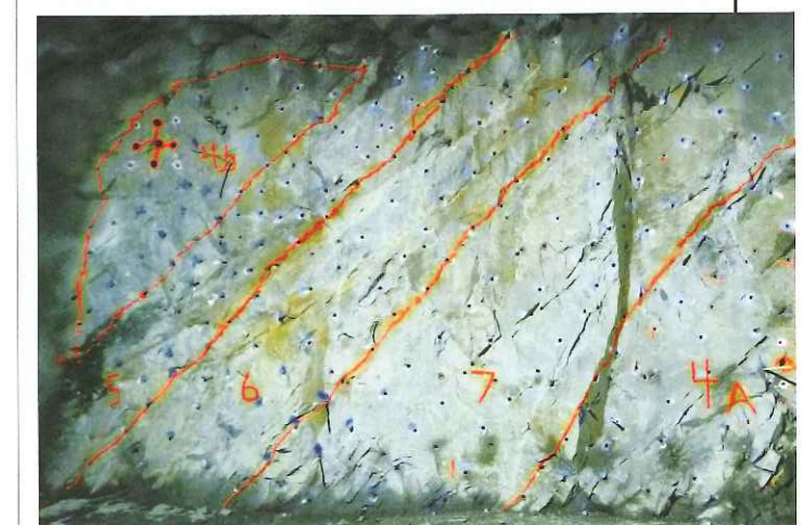
Below: Layout of blasts on 3m pillar face (red dashed lines represent approximate location of penstock)
