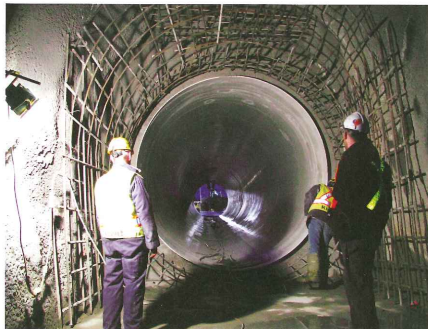
Below: A stretch of completed tunnel
