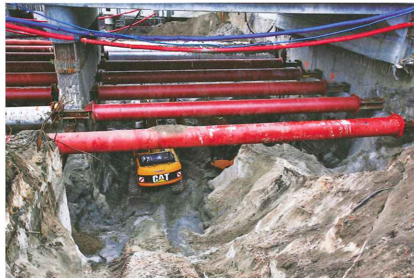
Above: Excavation of the tunnel approach on the river's far bank
