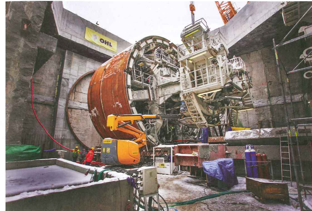
Left: The Martwa Wisla road tunnel in Gdansk, p.24
