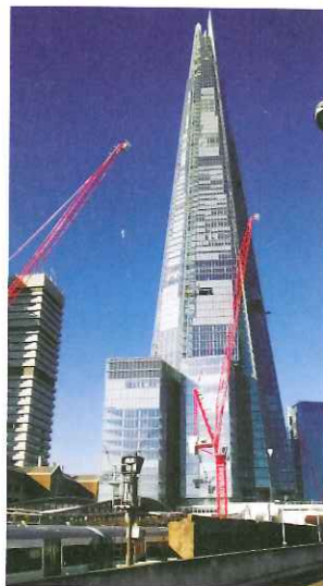
HTC cranes operating in London (not a Crossrail site)
