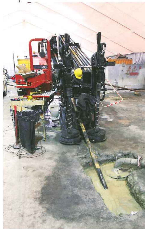
Left: A horizontal directional drilling rig
