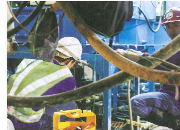
Above: Tight working conditions have been a challenge
