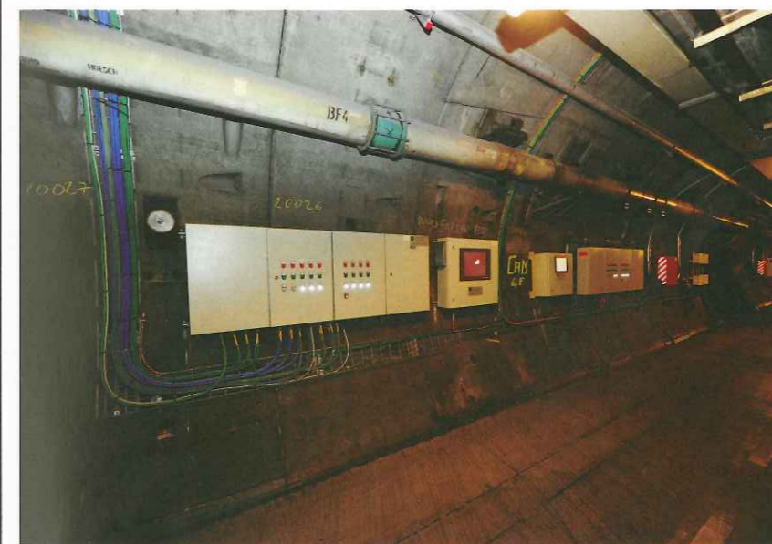
Above: Retro-fitted SAFE water-mist spray system in Channel Tunnel
