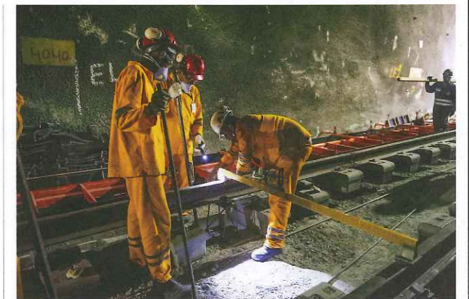
Top: Work underway on Oceanic Garden Station
