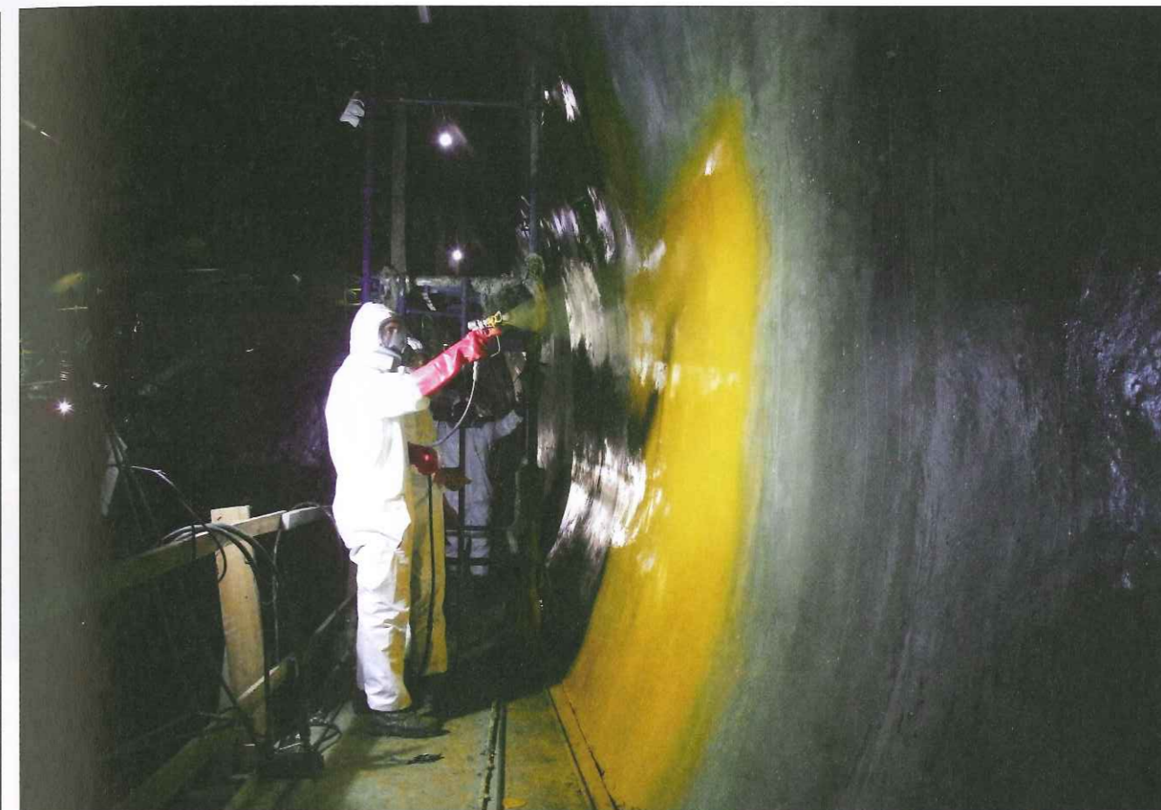
Above: Sprayed membrane application
