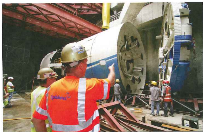
Above: A Robbins EPB is assembled at shaft bottom on CMC di Ravenna's C927 contract in Singapore
