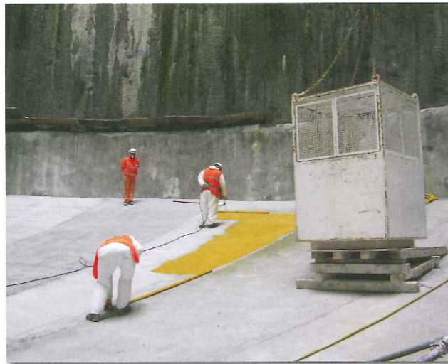
Above: Water-proofing application in stages
