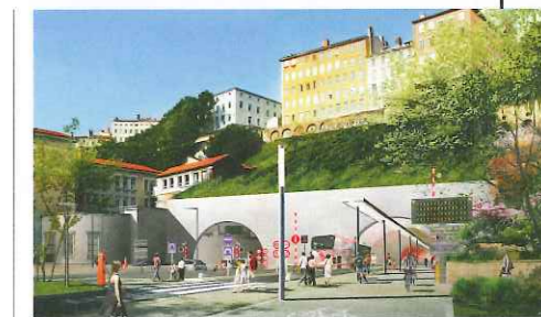
Right: Situation of the tunnel entrance in the side of the plateau
