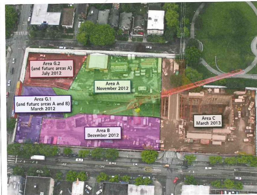
Above: Figure 1, the progressive handover of Capitol Hill station between contractors, which happened similarly at University of Washington station as well
