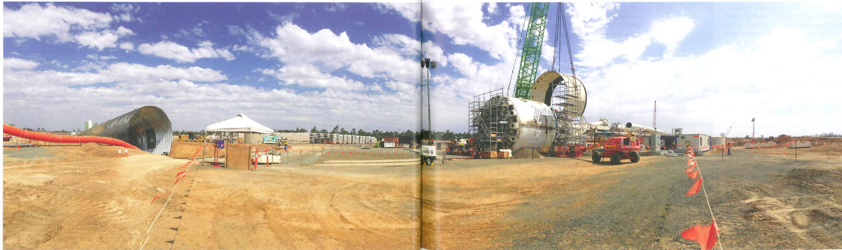
Below: Hybrid currently under assembly, that has been designed as explosion proof for a coal mine
