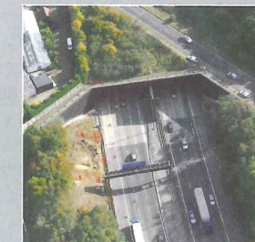
Bell Common Tunnel, London
