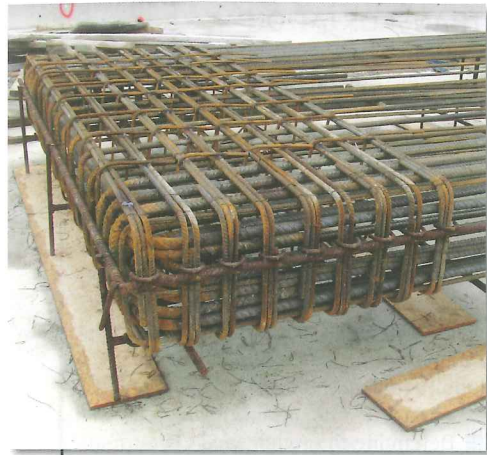
Left: Immersed element reinforcement
