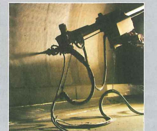
Groene Hart Tunnel, Netherlands
