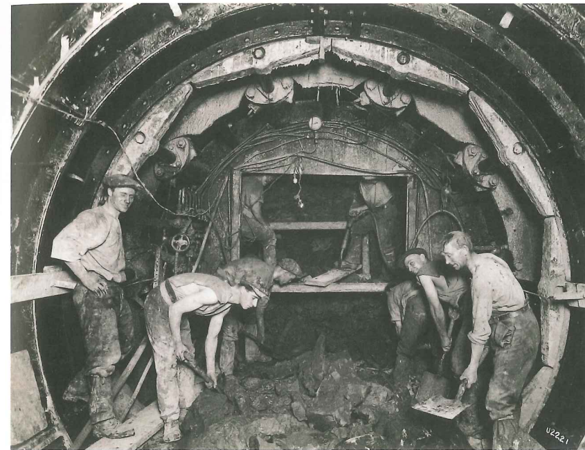
Above: Excavation work on the Northern Line TFL
