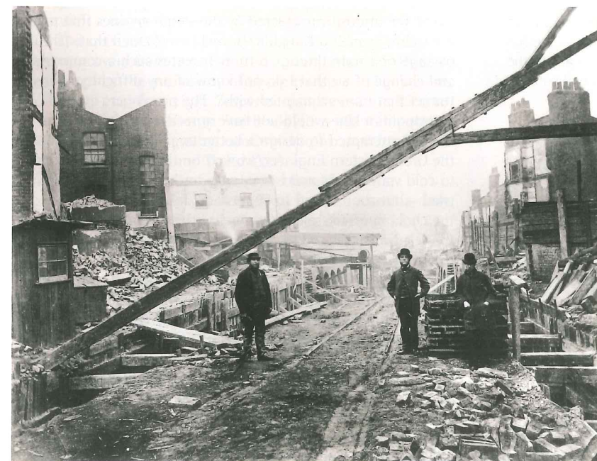
Below: Cut and cover on the Metropolitan Railway extension to Kensington. Work begins on the retaining walls TfL
