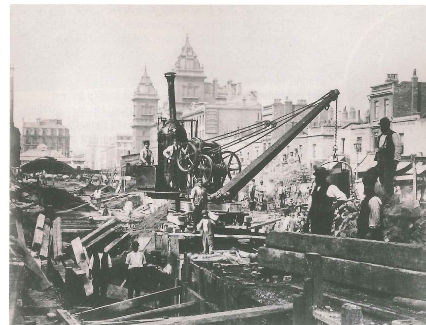
Above: Metropolitan Railway work at Praed Street, Paddington TFL
