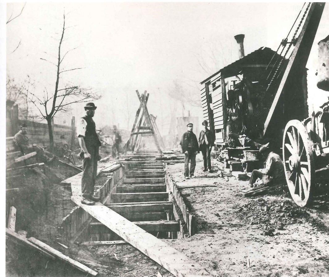
Below: Cut and cover on the Metropolitan Railway extension to Kensington. Work begins on the retaining walls TfL
