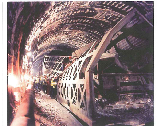
Above: A wrecked carriage following the 1996 Channel Tunnel fire
