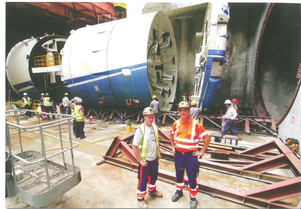
Above: Five Robbins mixed ground EPBMs are excavating portions of Singapore's Downtown Line, a massive project using 29 TBMs simultaneously
