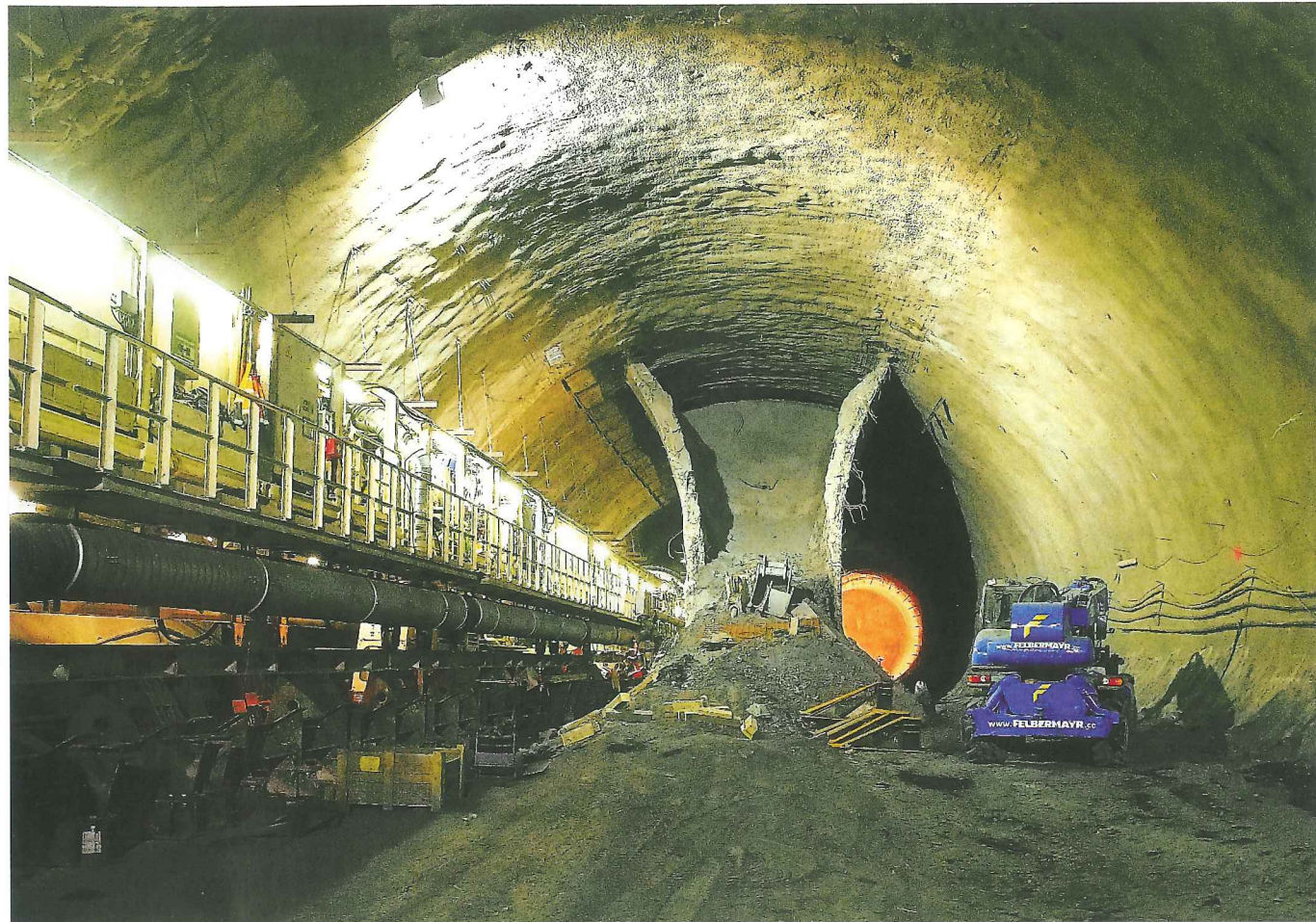
Above: Reusable steel structure with Tonda at Cervený vrch
