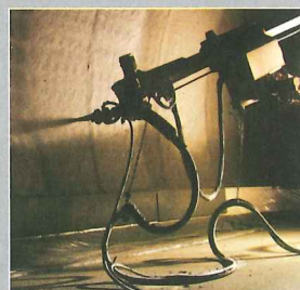
Groene Hart Tunnel, Netherlands
