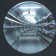
CITY EAST CABLE TUNNEL, NSW
