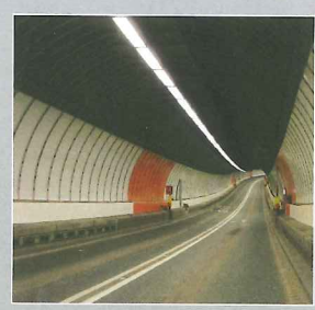
Clyde Tunnel, Scotland
