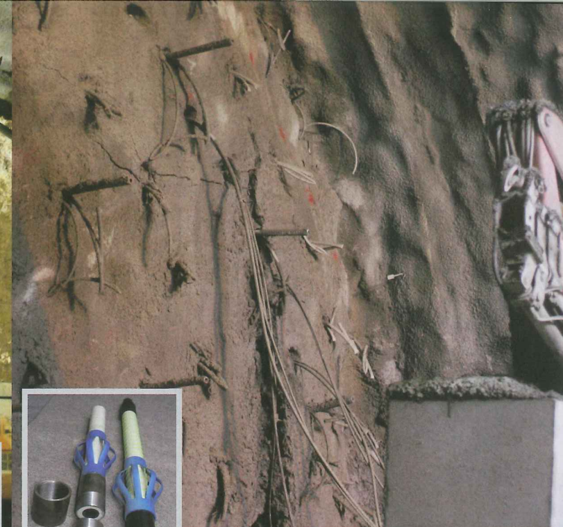
Glass Fibre (GFRP) profiles for cost effective, high performance face consolidation
