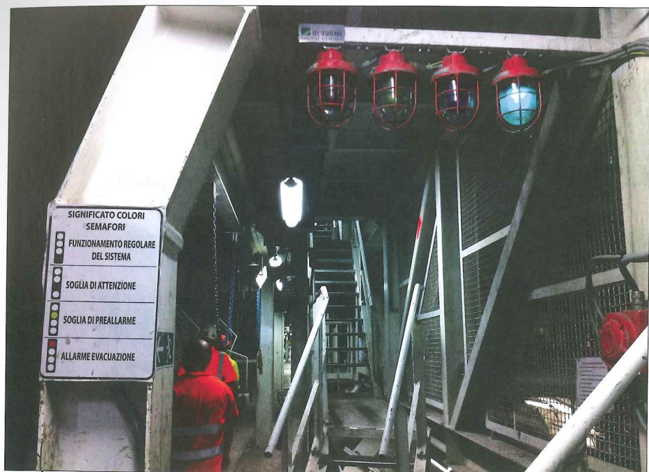
Above: A traffic light-style warning system for methane gas in the Appenines
