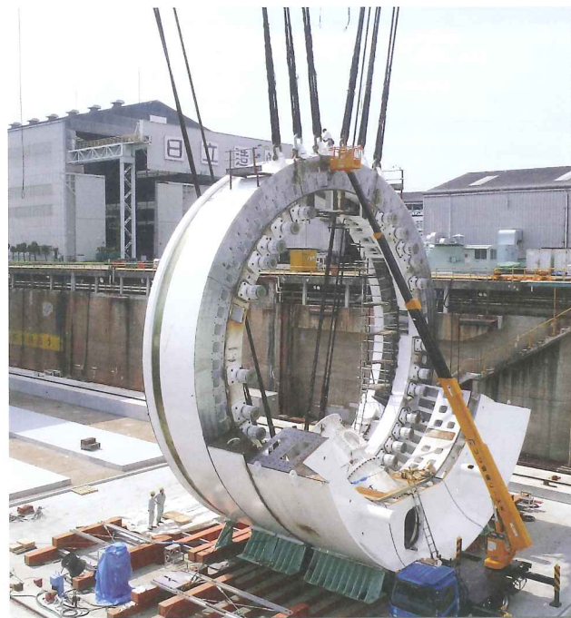
Above: Assembly of the 17.5m diameter TBM for Alaskan Way
