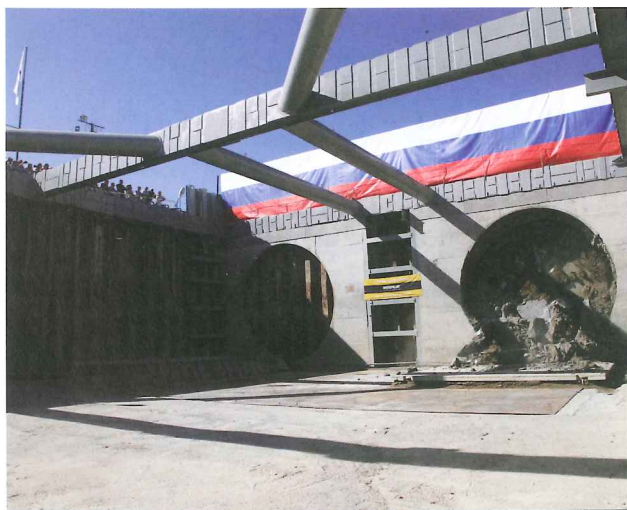
Above: The Caterpillar TBM broke through on the Omsk Metro
