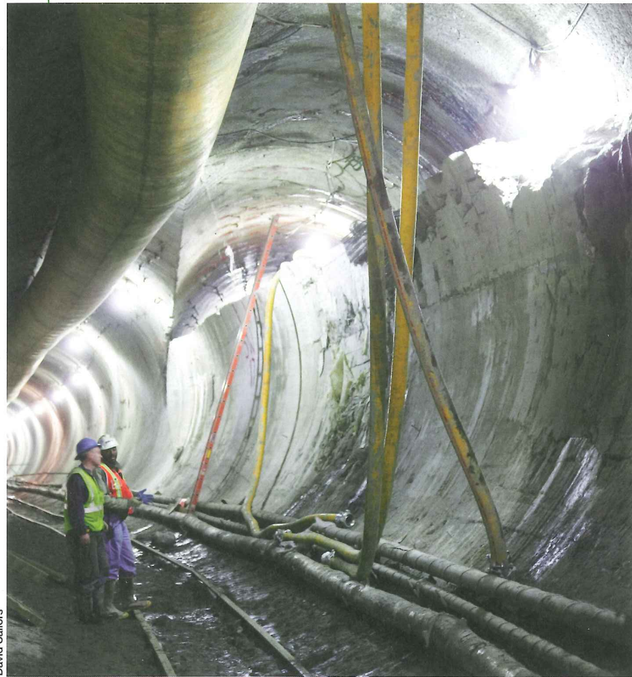
Above: Workers inspect segmentally lined running tunnels
