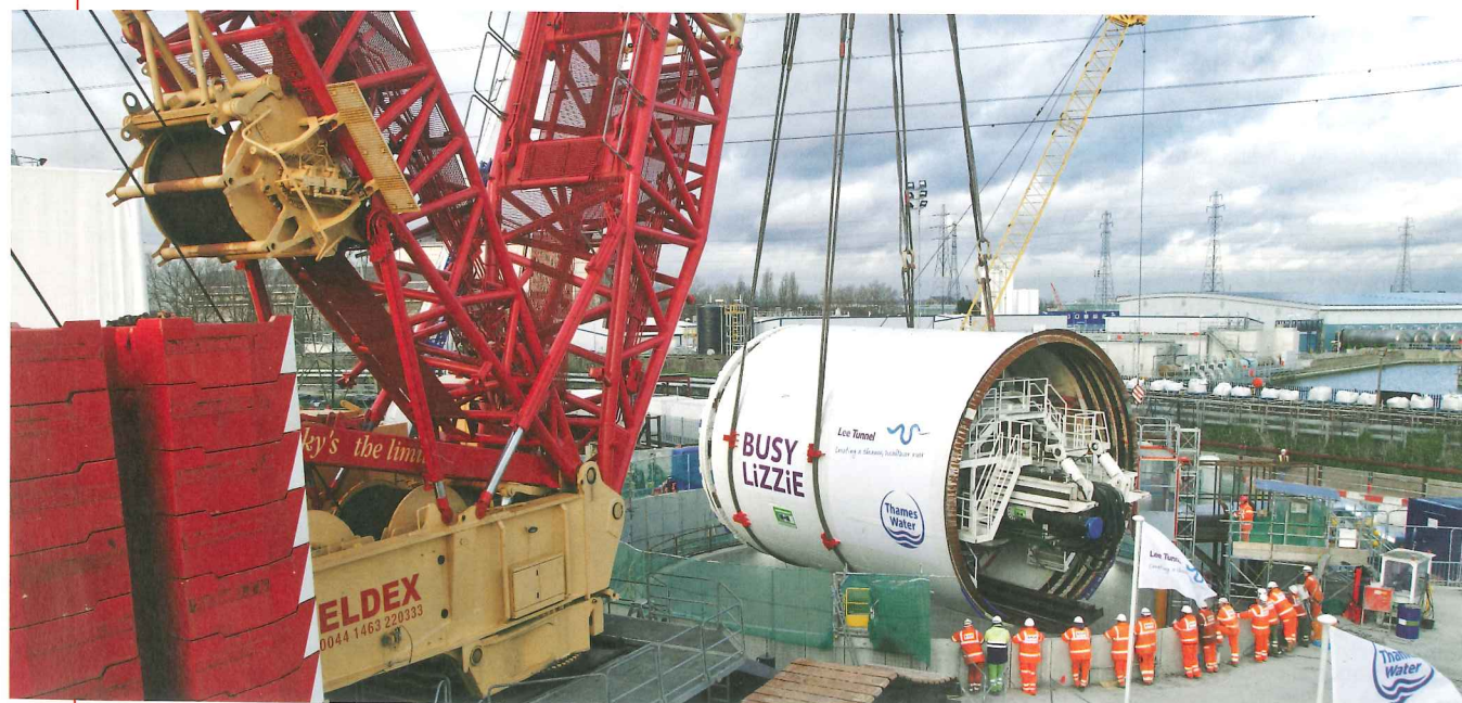
Below: Lowering the TBM
