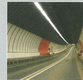
Clyde Tunnel, Scotland
