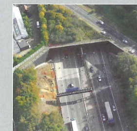
Bell Common Tunnel, London
