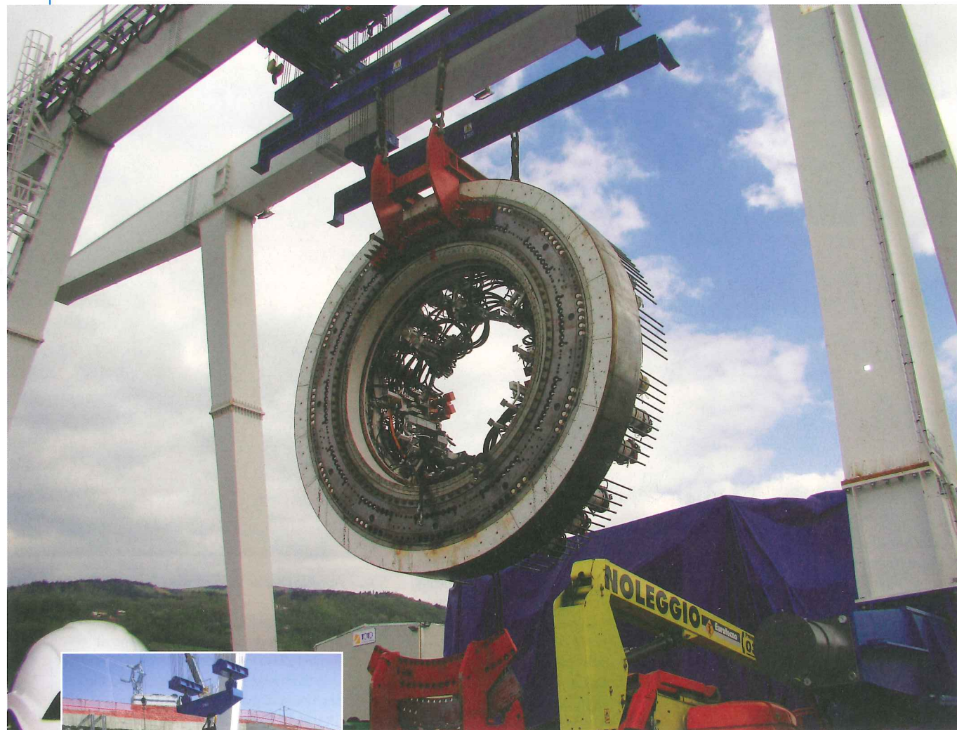
Above and left: Assembly of the Sparvo TBM by contractor Toto and manufacturer Herrenknecht at a section of the A1 Highway between Florence and Bologna, Italy
