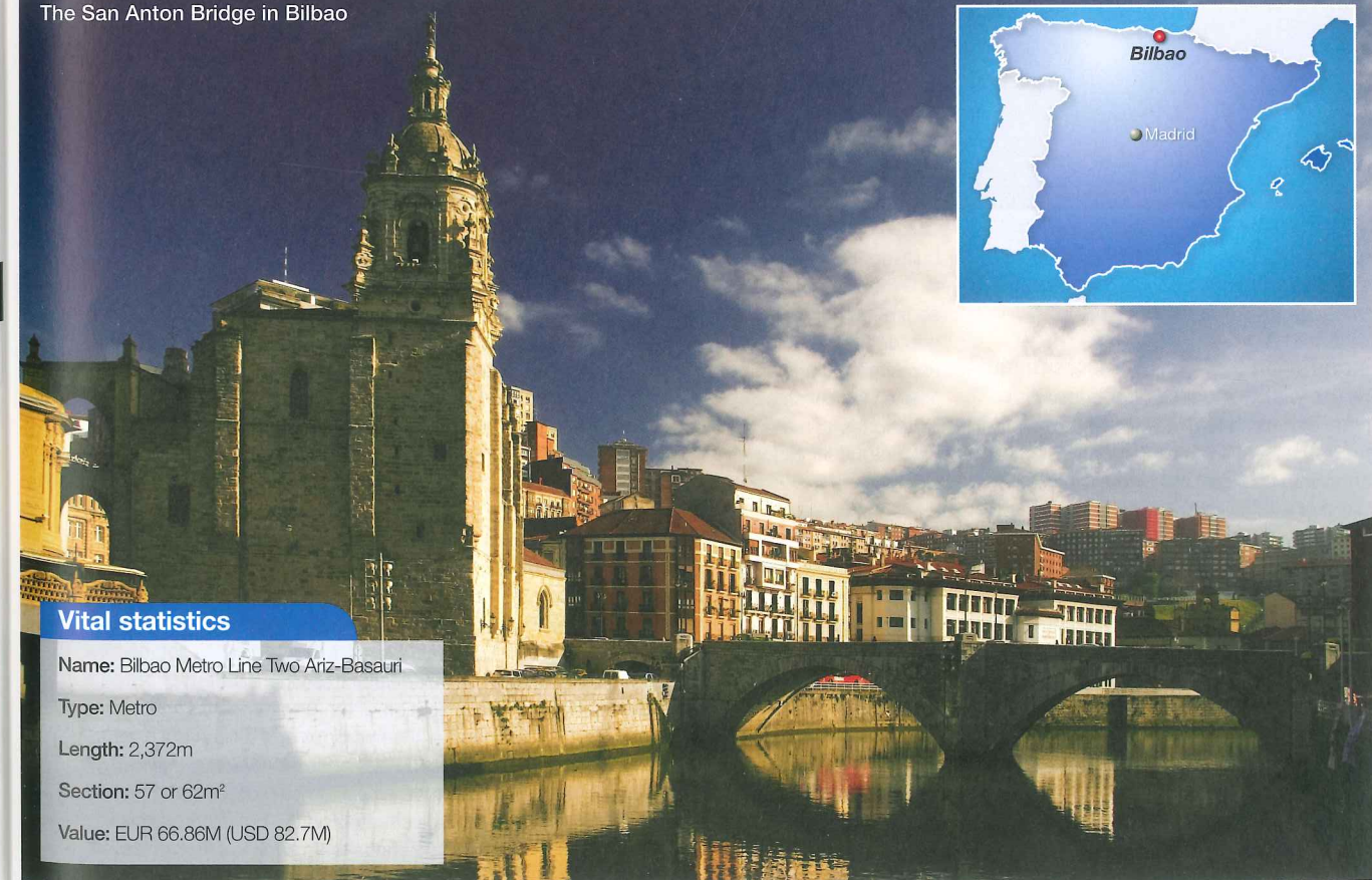
The San Anton Bridge in Bilbao
