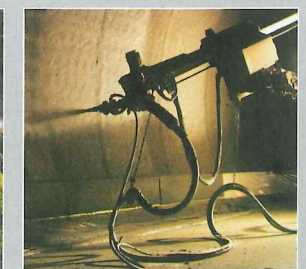
Groene Hart Tunnel, Netherlands
