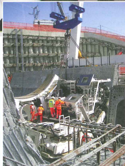
Above and left: Assembly of the Sparvo TBM by contractor Toto and manufacturer Herrenknecht at a section of the A1 Highway between Florence and Bologna, Italy
