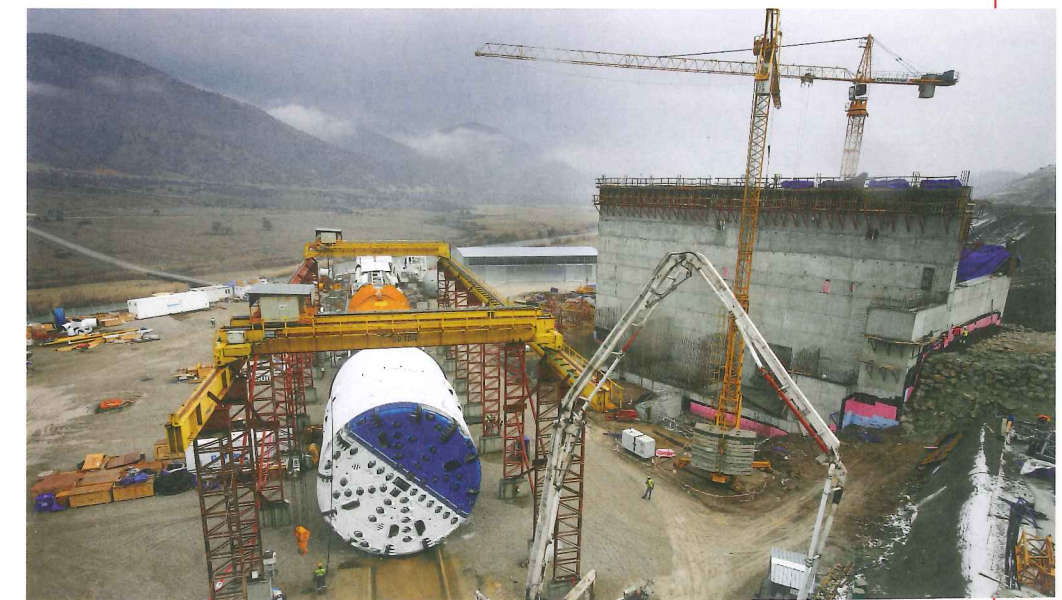
Below: Machine assembly
