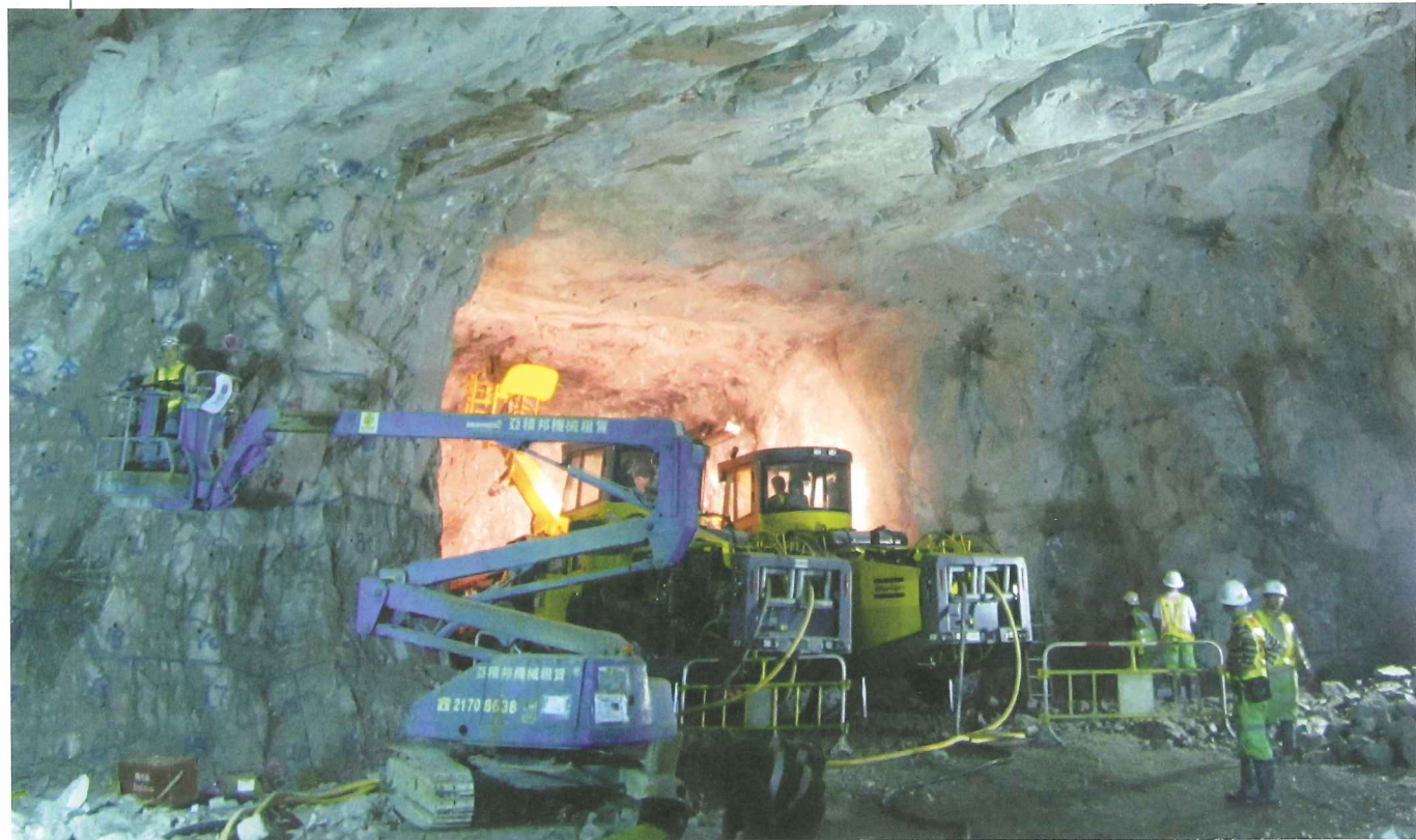
Above: Excavation work on the West Island Line in Hong Kong
