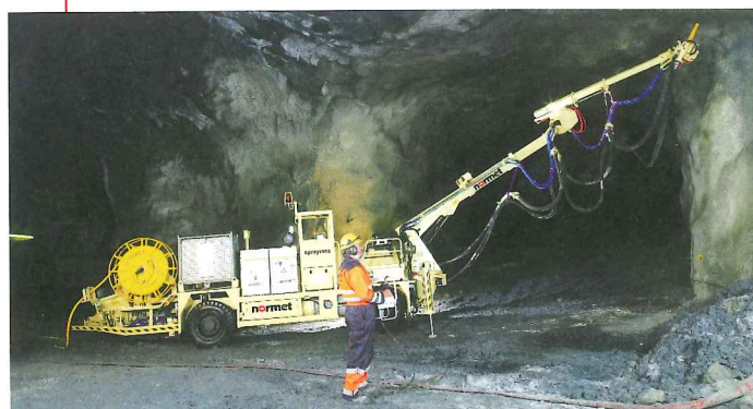
Below: Normet Spraymec 8100 VC 1 in operation
