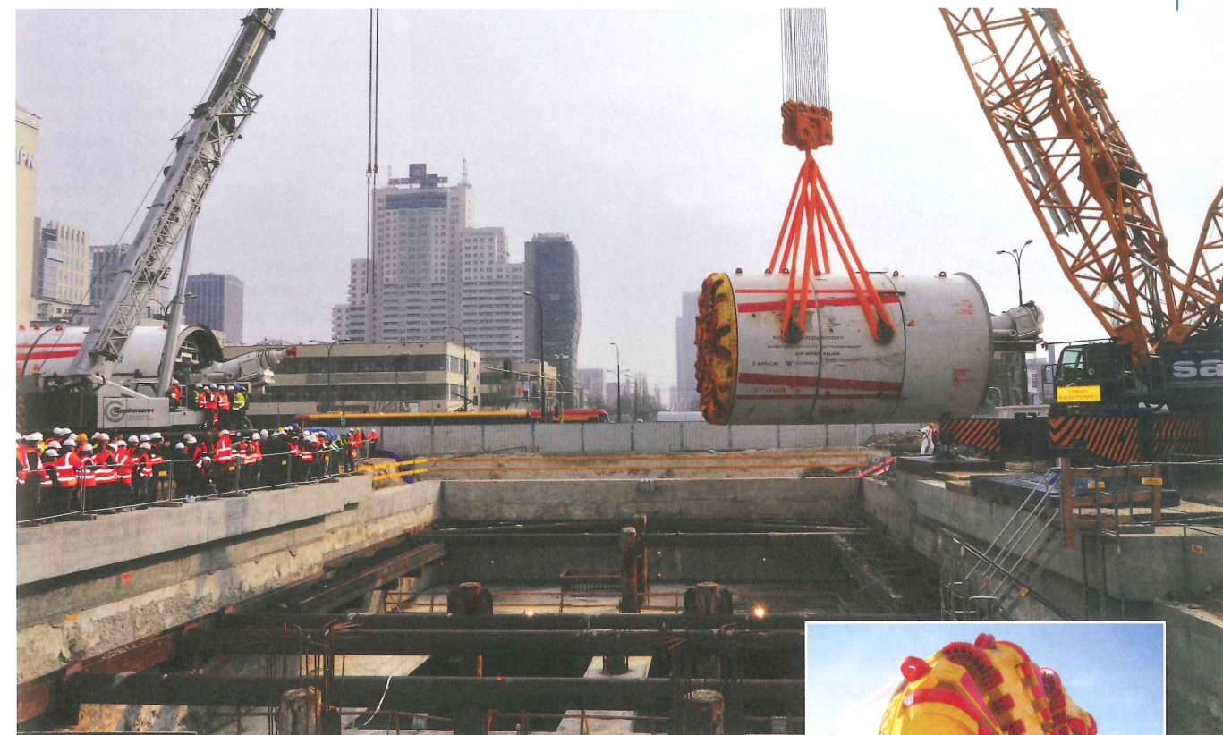
Above: The machine being lowered down the shaft to bore the second metro line Right: Herrenknecht manufactured the four EPBMs for the project. The machines have a diameter of 6.3m, giving a finished tunnel i.d. of 5.4m
