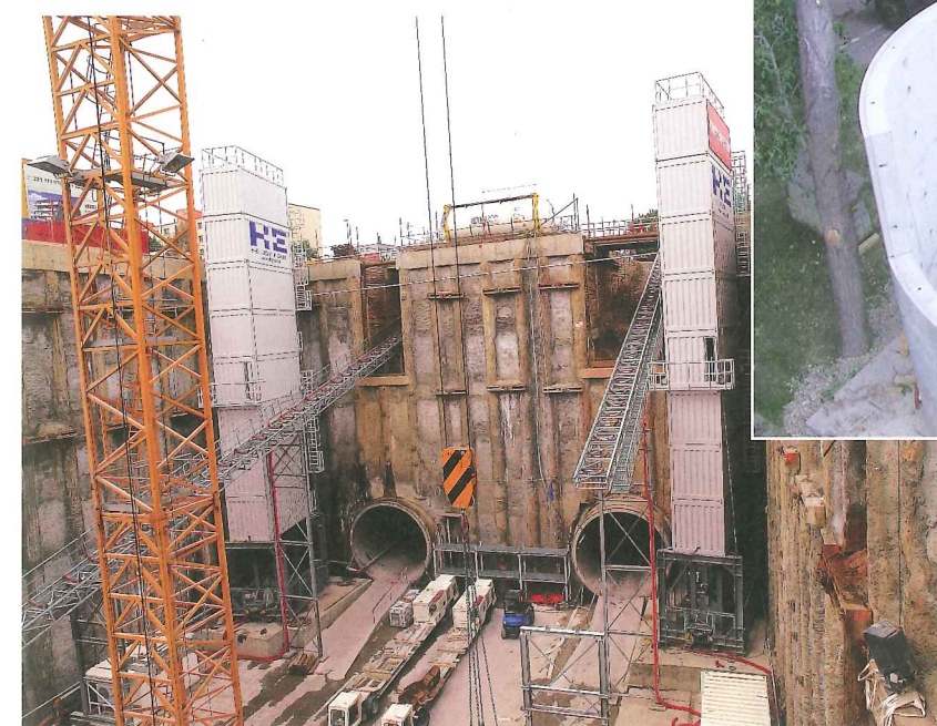
Above: The E2 site with conveyor belt-supporting structures under construction
