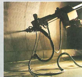
Groene Hart Tunnel, Netherlands
