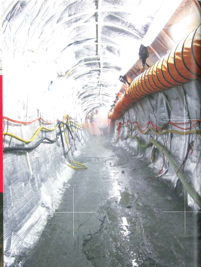
| MTRC WEST ISLAND LINE CONTRACT 703 | HONG KONG → Ground frozen tunnel for the removal of underground obstruction
