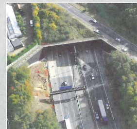
Bell Common Tunnel, London
