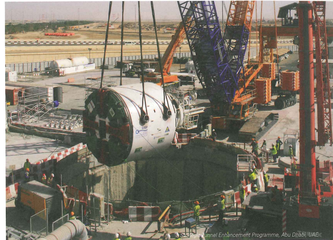
Strategic Tunnel Enhancement Programme, Abu Dhabi, UAE
