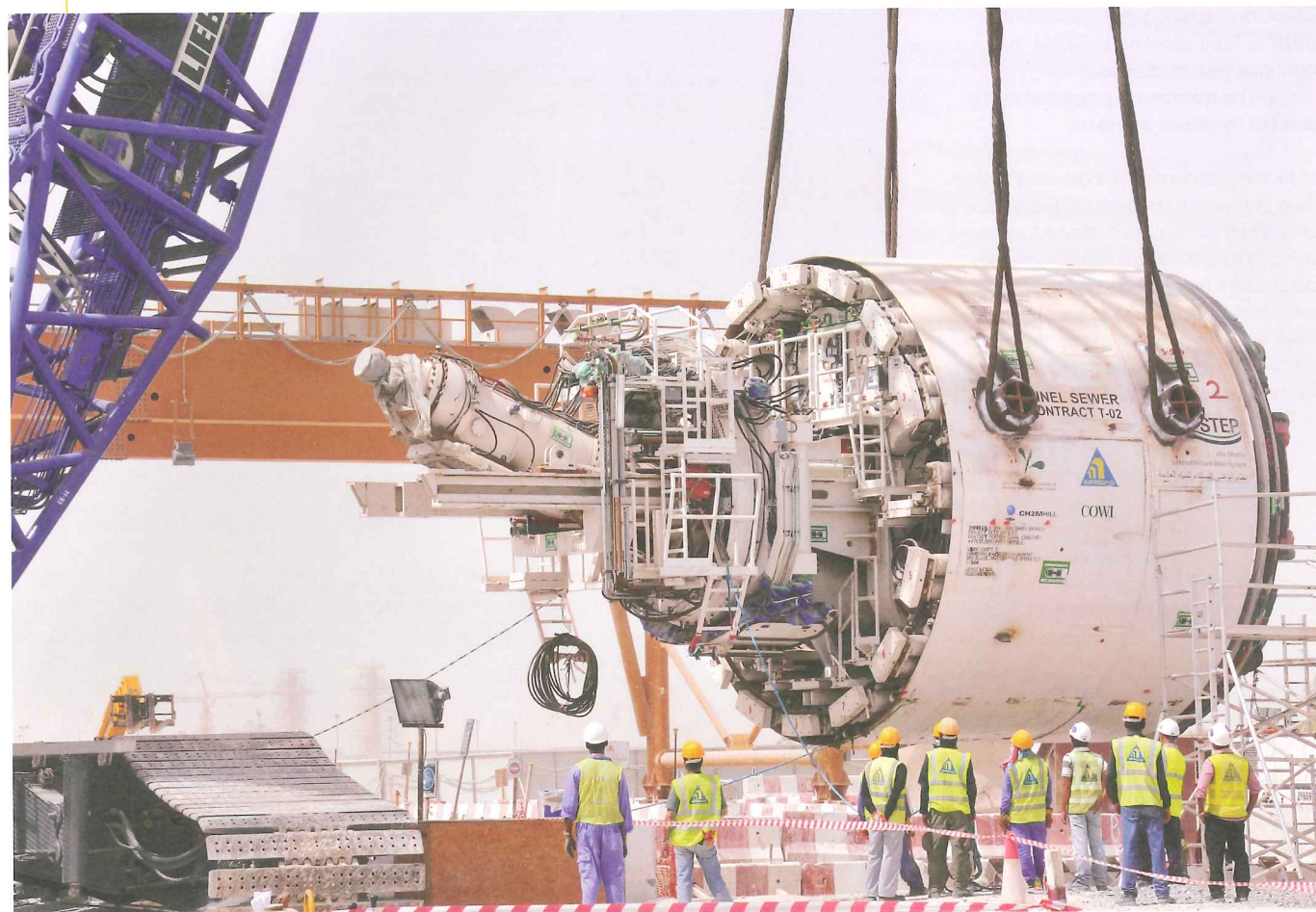
Above: The third EPBM is lowered into its launch shaft on contract T02
