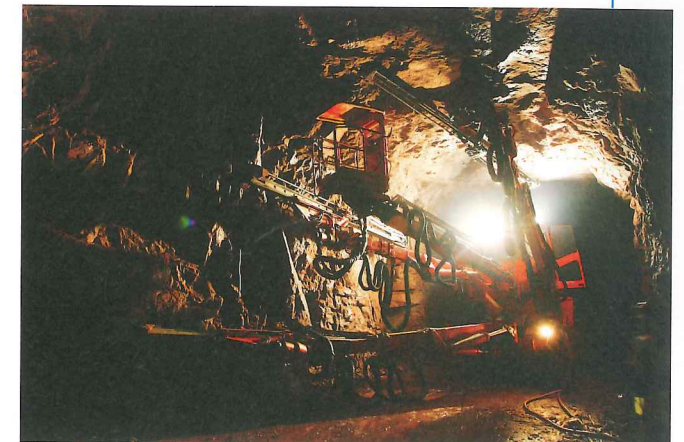
Above: Excavation on the Lansimetro (West Metro) in Helsinki
