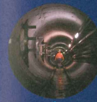
CITY WEST CABLE TUNNEL, NSW
