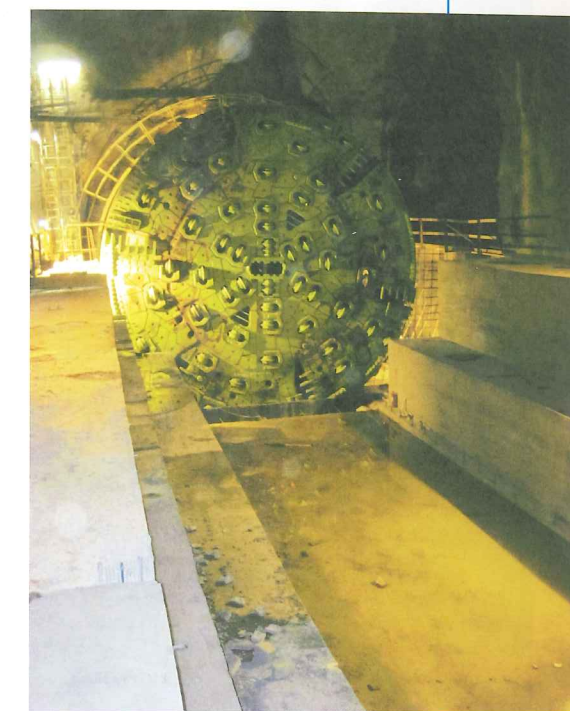
Above: A TBM mining the Hallandsas railway tunnel.
