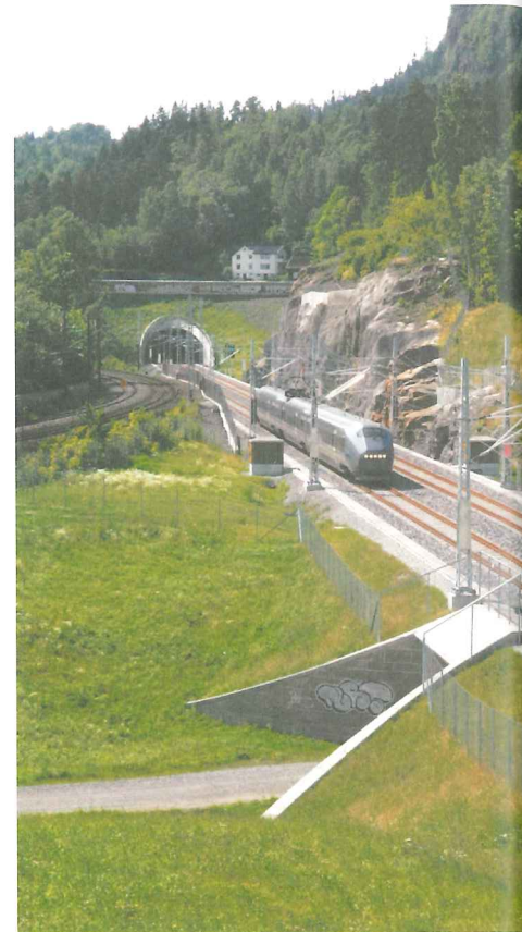
Above: Rail is one five main demands for tunnelling in Norway
