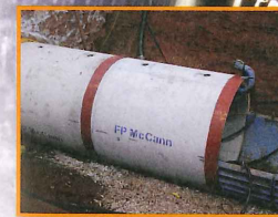
Jacking Pipes
