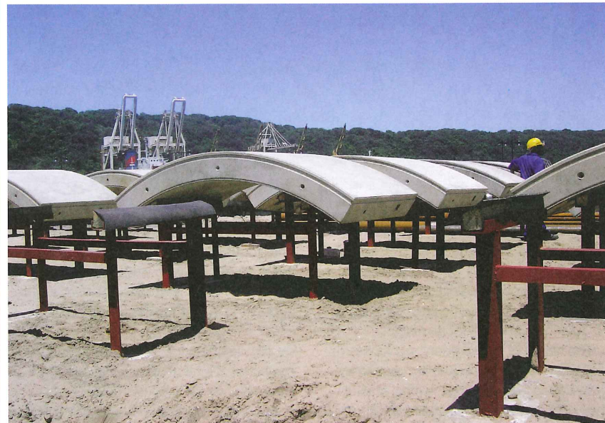
Above: Segments supported on frames while curing to full strength
