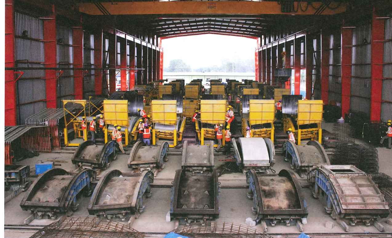
Peenya precast factory makes use of CBE moulds. Segment production is subcontracted to YaLi
