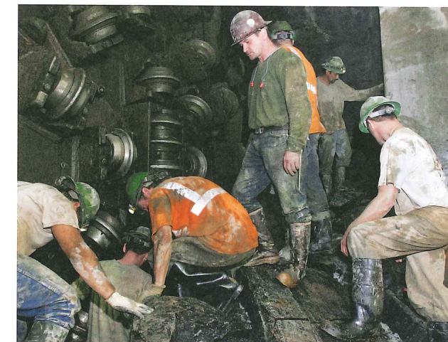
Above: Breakthrough at Second Avenue (photo courtesy of MTA)
