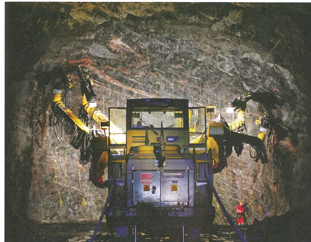
Above: The Boomer XE4C rig at the tunnel face of Hede-Alvängen
