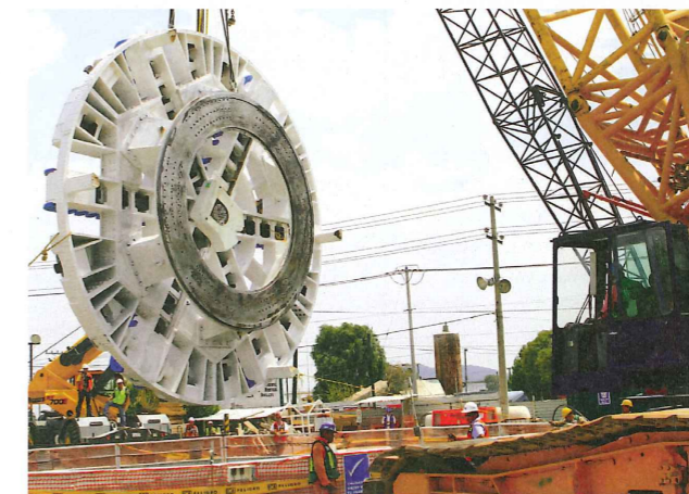
Right: Cutterhead assembly
