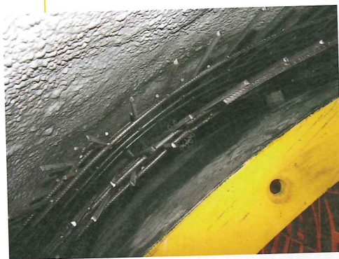
Above: Proximity of reinforcement wire etc to the membrane may result in accidental penetration; Below: Some planned penetration of the membrane can be allowed if sealed as with reinforcing mesh
