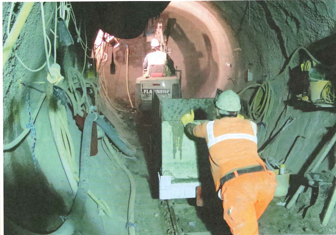
Above: Connecting tunnel for the Dorchester Hotel service link
