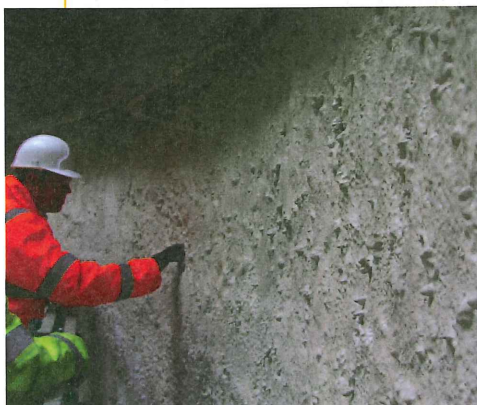
Left: Examining the sprayed membrane applied in the Hampton pump-out shaft
