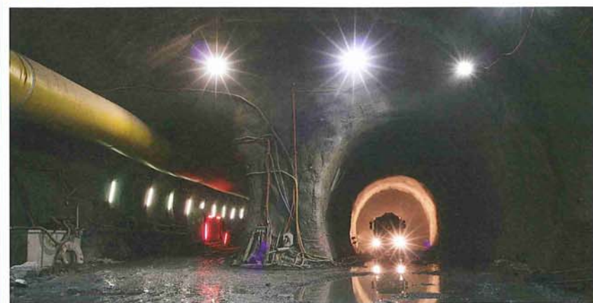
Above: Central access cavern from which main drives begin
