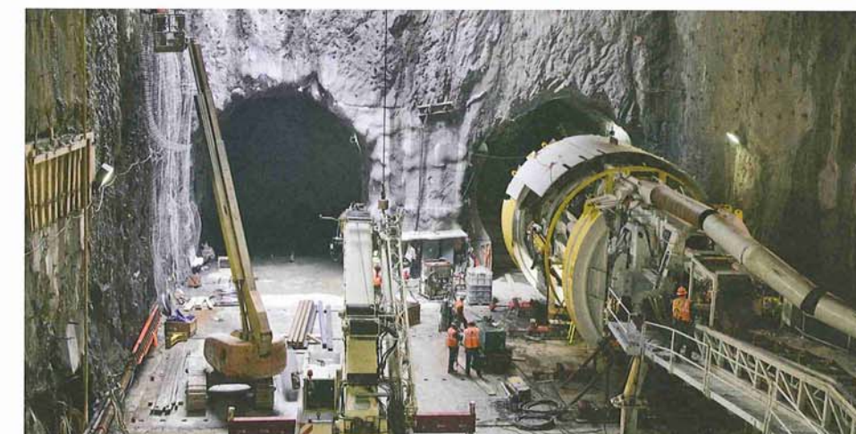
Above: Completion of the West tunnel was a significant milestone
