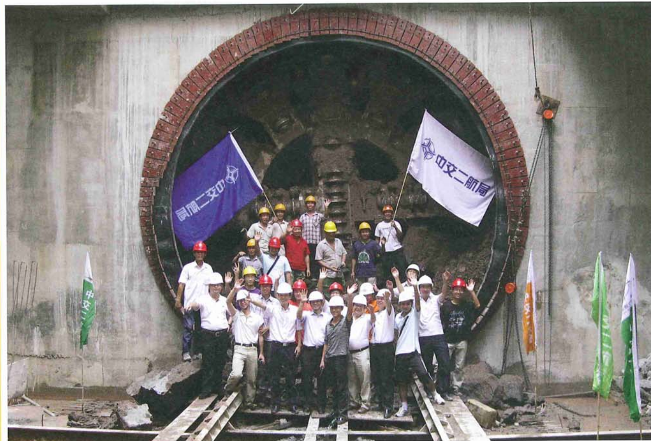
Above: The Robbins EPBs at Guangzhou Metro broke through ahead of schedule, despite facing challenges including low tunnel cover and layered soft ground with rock.
