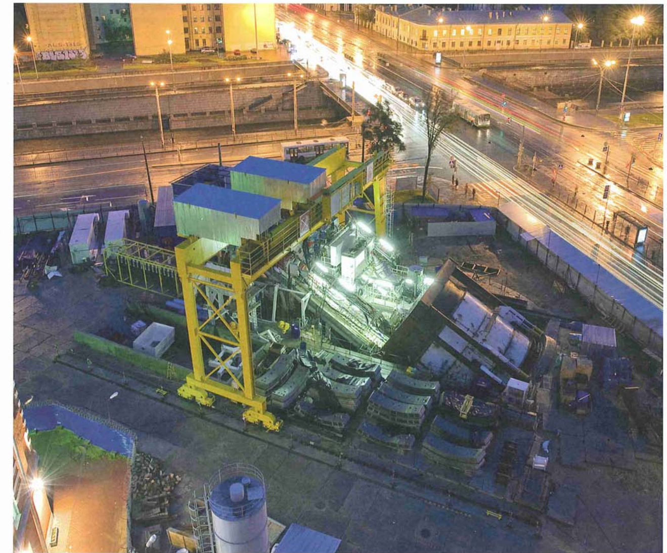
Above: A new escalator shaft in the heart of St. Petersburg
