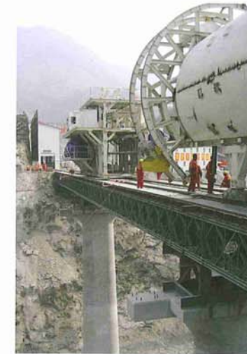
Above, left: Both Robbins machines were walked into 2,000m launch chambers, with the back-up and muck haulage systems starting from bridges across a deep valley; Above, middle: Ground support in the high cover tunnels consists of ring beams, wire mesh, and rock bolts, with the McNally support system optional in unstable ground; Above, right: Final lining with concrete is taking place behind both Robbins TBMs at West Qinling
