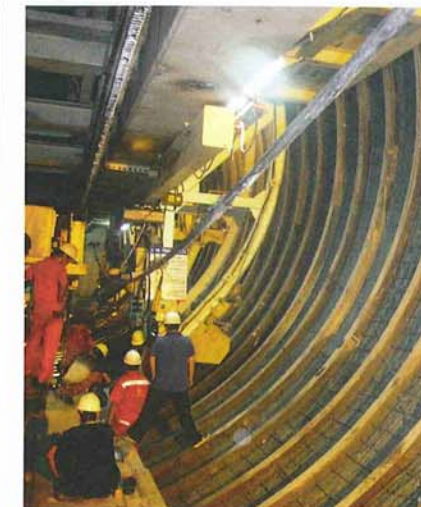
Above, left: Both Robbins machines were walked into 2,000m launch chambers, with the back-up and muck haulage systems starting from bridges across a deep valley; Above, middle: Ground support in the high cover tunnels consists of ring beams, wire mesh, and rock bolts, with the McNally support system optional in unstable ground; Above, right: Final lining with concrete is taking place behind both Robbins TBMs at West Qinling
