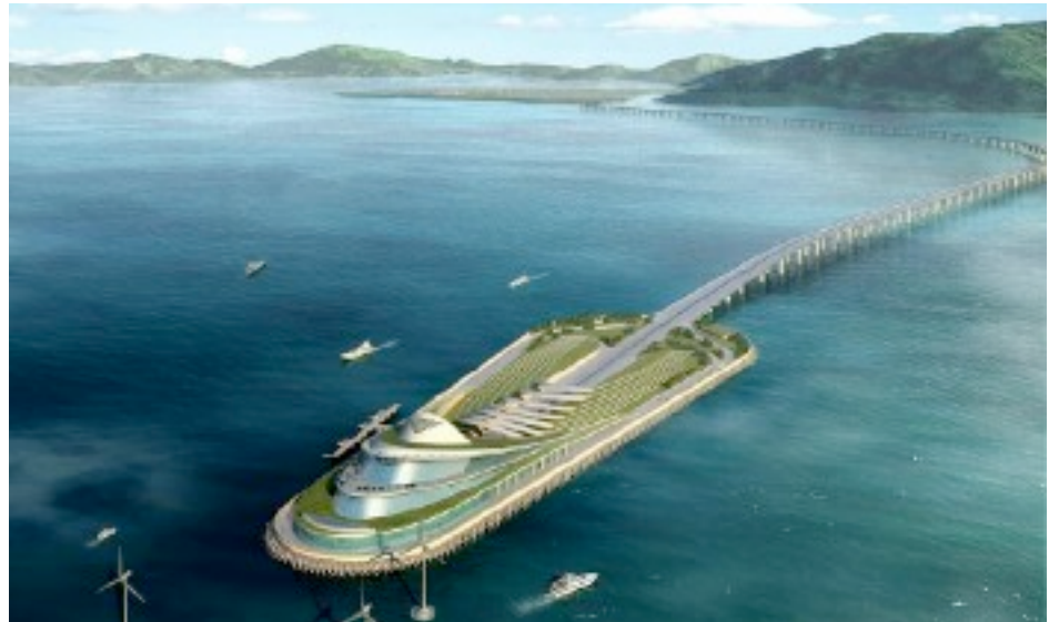
Above: The link with switch from the elevated bridge to the immersed tube tunnel via an artificial island
