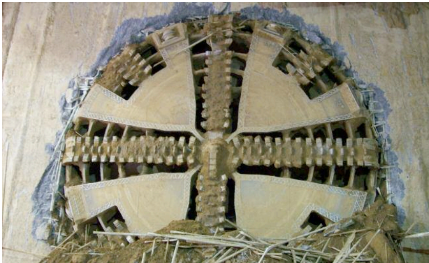
Left: Breakthrough of one of the 6.64m diameter EPBM
