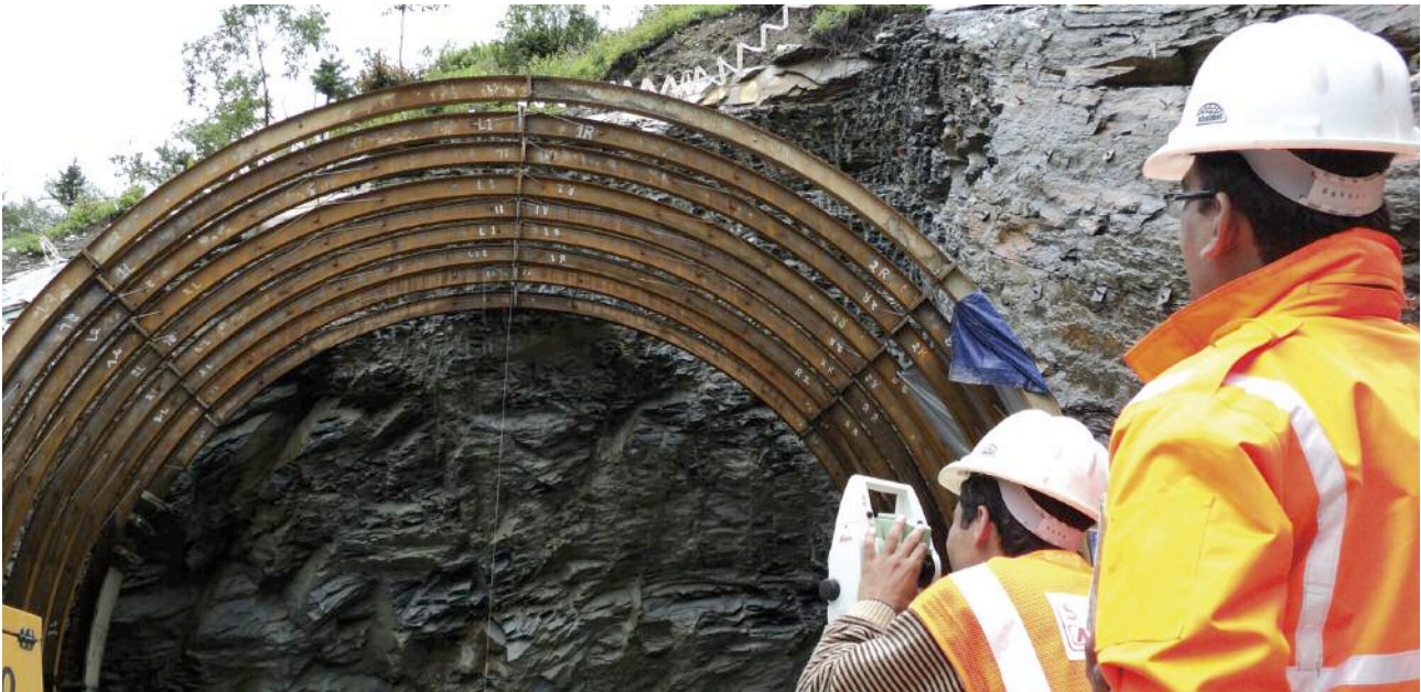
Above: Monitoring the steel section; Below: Over and under break in the rock excavation
