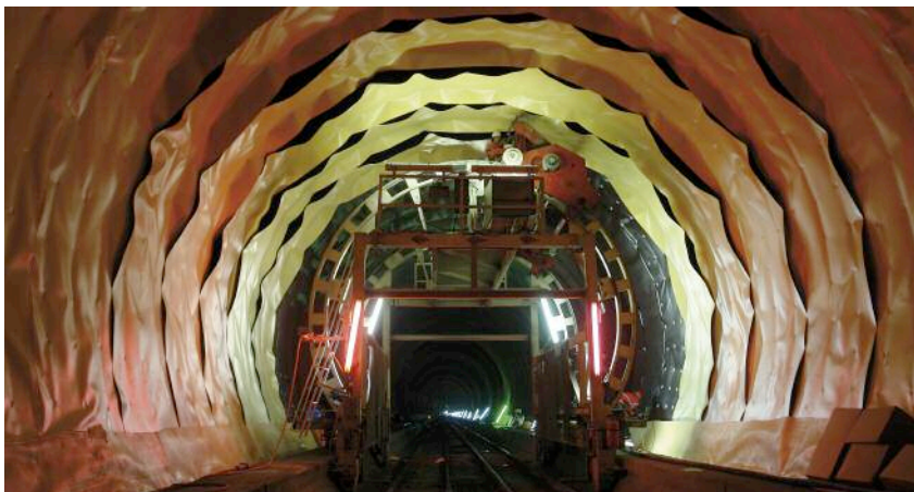
Left: Impermeable membrane being installed for the lining formwork Below: Rescue sequence for the TBM trapped in disaggregated ground
