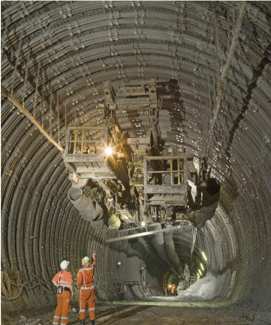
Above: Close spacing of the sliding support circles on the northern drives at Sedrun
