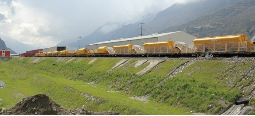
Left, top and bottom: The multi-wagon concreting train
