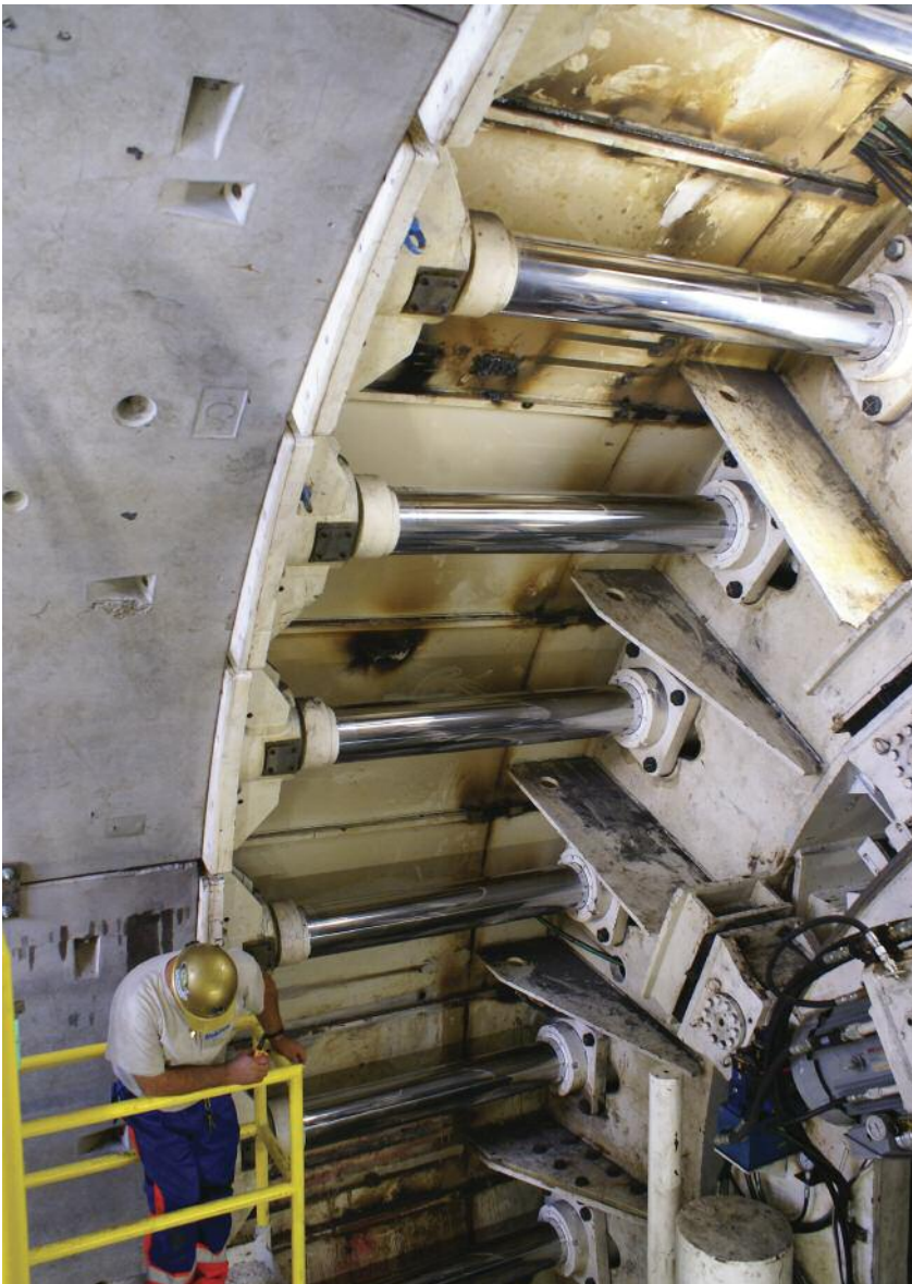
Left: The EPB TBM installs a segmental lining as it excavates the Line 12 tunnel
