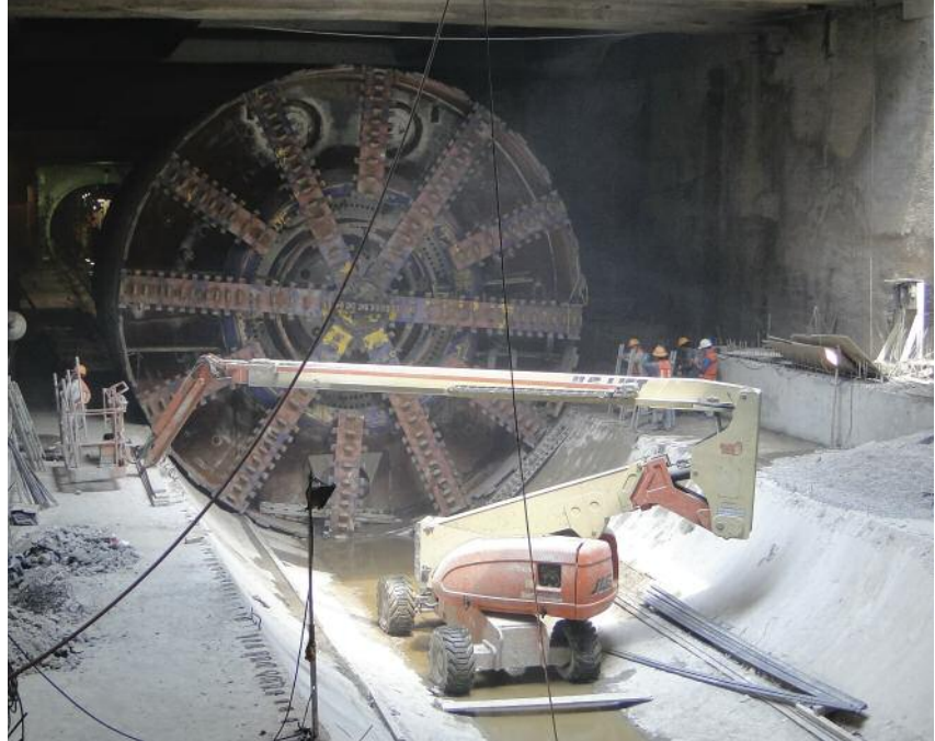
Right: The Robbins EPB TBM after its breakthrough to Mexicaltzingo Station
