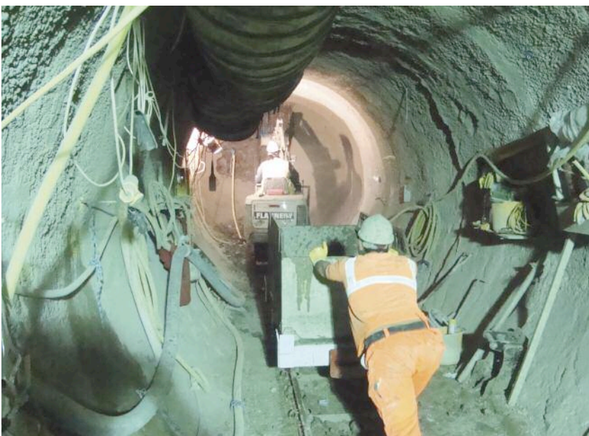
Above: Excavation and mucking during tunnel excavation: 1.5T excavator and 1T hand-pushed skip on rails
