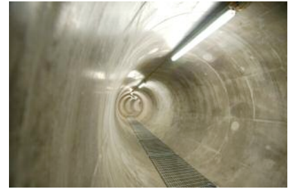
Above: The finished tunnel lining
