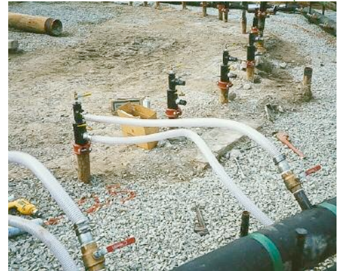
Above: Ground freezing on San Diego South Bay Ocean Outfall project
