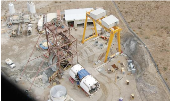
Left: Front shield pieces of the TBM are ready to be lowered into the assembly chamber at Lake Mead
