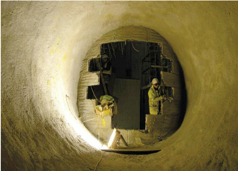
Above: Looking into the 45 Park Lane shaft following Masterseal application
