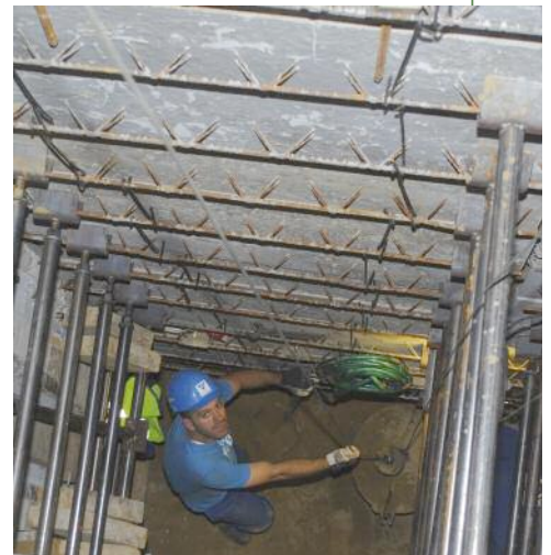
Above: Busy excavating the wall slots
