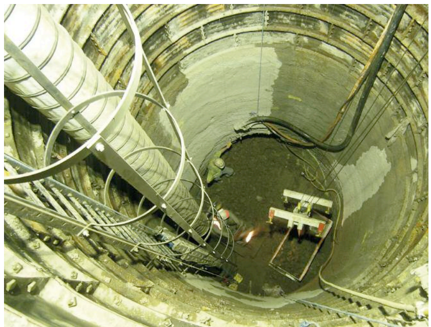
Above: The Dorchester shaft under construction using steel liner plates
