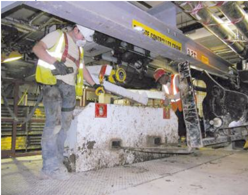
Left: The working area at the top of The Dorchester shaft
