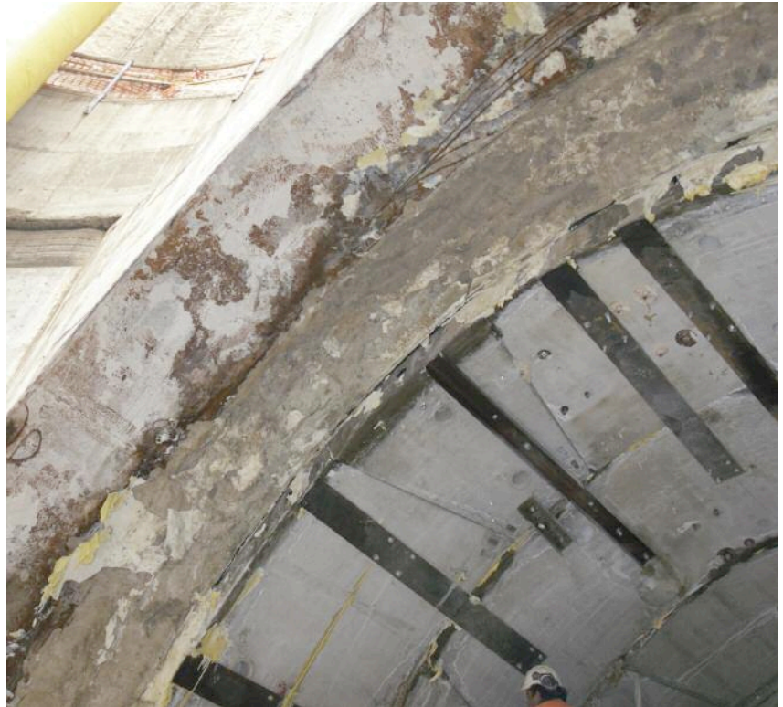
Above: The whole annular space has been filled with the two-component material. Left and below left: Extraction of a segment and presence of the two-component material in the annular space.
