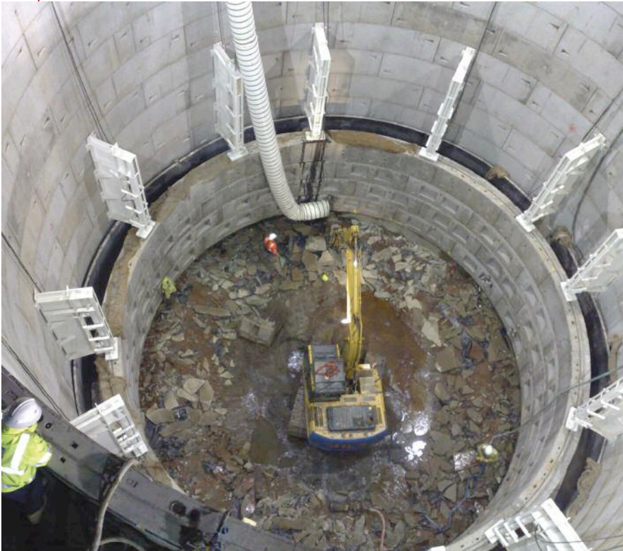
Above: Building the inner caisson in T1
