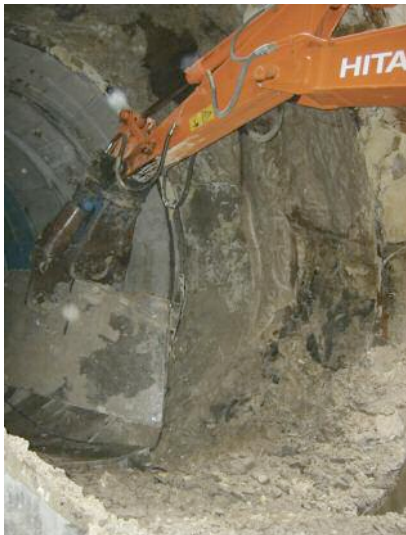
Above: The whole annular space has been filled with the two-component material. Left and below left: Extraction of a segment and presence of the two-component material in the annular space.
