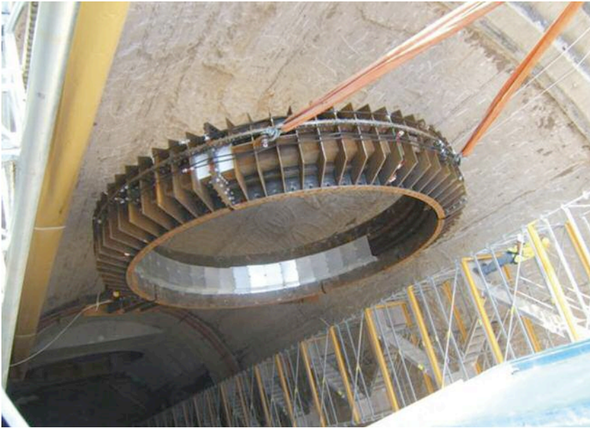
Left: The 2-seal ring can be reused in other projects of the same dimension and characteristics
