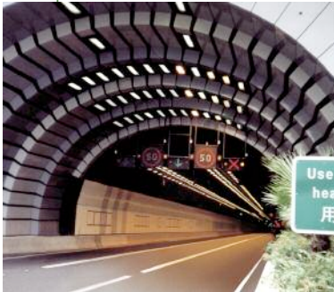
Above, left: Thorlux lighting near the portal of a road tunnel with Scanlight control from P Ducker Systems; Above, right: Quickly noticeable and understandable signage is vital for both normal traffic control and incident management [Siemens press picture]
