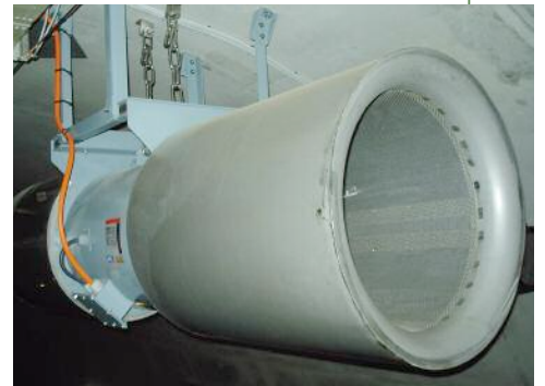
Above: Actuation of ventilation dampers is an important element of ventilation for smoke control and fire oxygen starvation [Photo: HBI Haerter]
