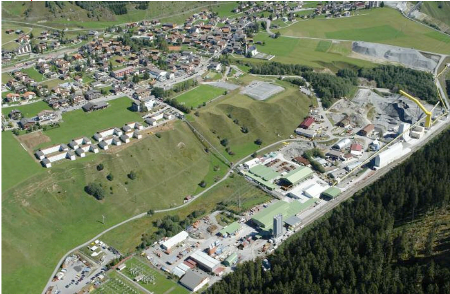
Left, top to bottom: Schematic of the Sedrun section of the Gotthard Base Tunnel with access routes; Surface accommodation and other facilities near Sedrun; Sedrun shaft bottom with hoist cages
