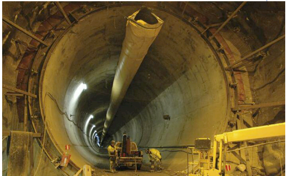
Above: Pre-cast segmental lining seen from the TBM erection chamber
