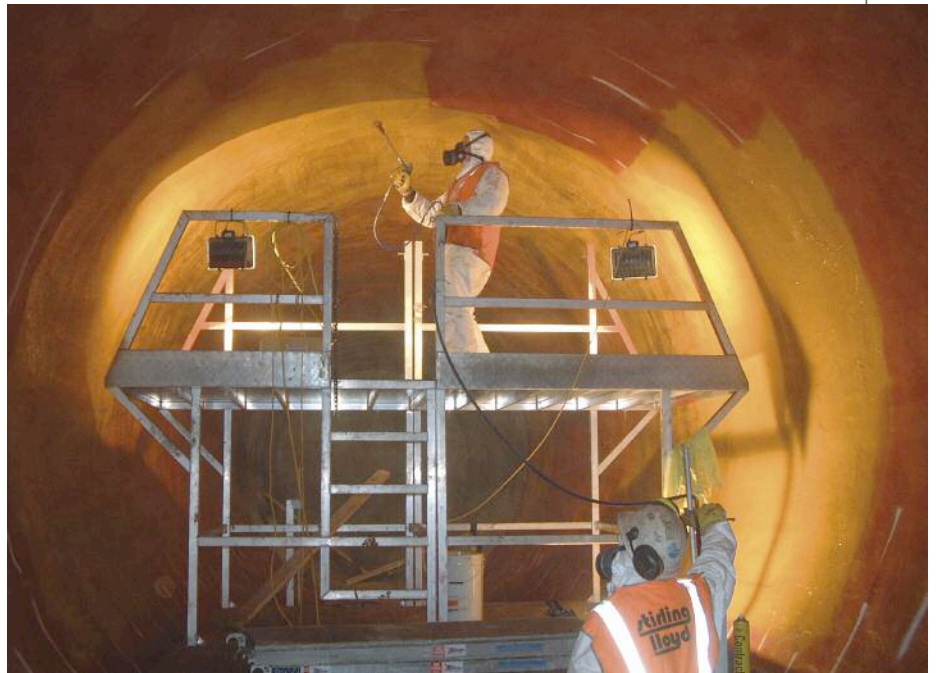
Above: A custom-built platform give operators better access in the Thames Water Ring Main extension
