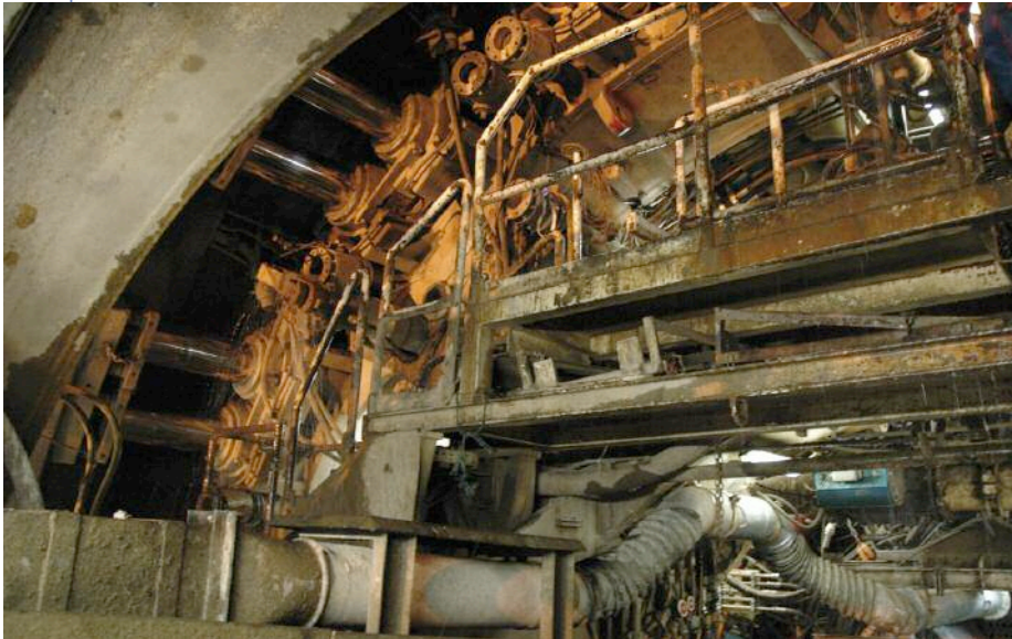
Above: Thrust rams within the Herrenknecht TBM shield
