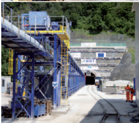
The belt storage at the Aica / Aicha-Mules / Mauls tunnel portal.
