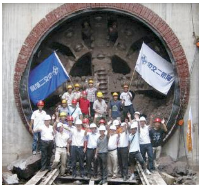
Above: The first 6.3 m diameter Robbins EPB broke through into the Xilang Station site in August 2009.
