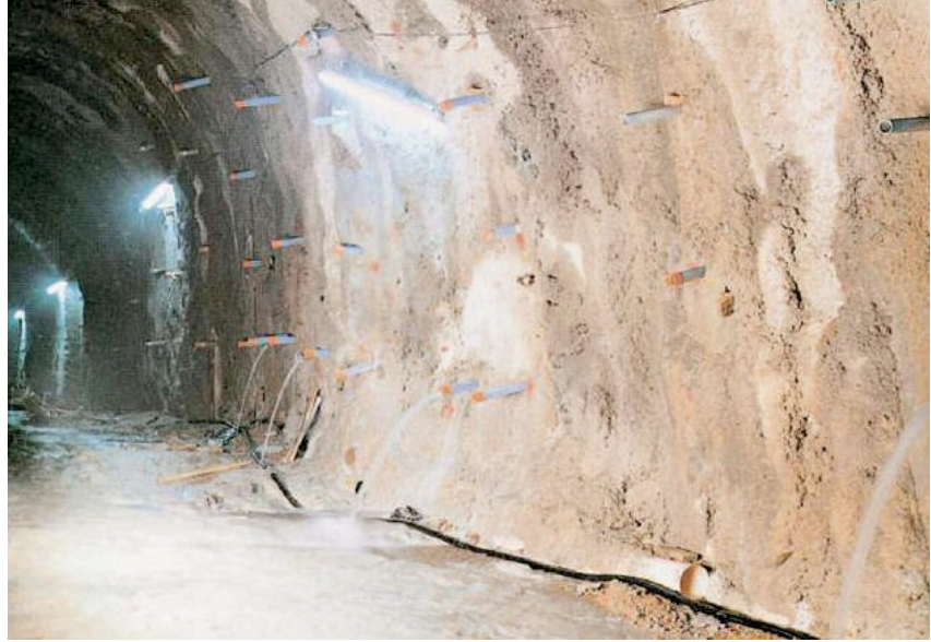
Above: Image 7 - Sireg drainage pipes with slots used to dewater soft soil around a tunnel excavation to prevent ground degradation
