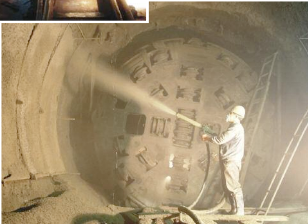
Left and Below: The 4.8m TBM is excavating mixed ground including soil and hard rock
