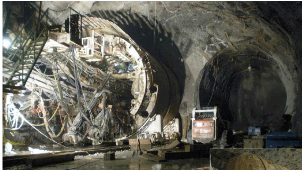
Above/Right: The 6.7m diameter TBMs will bore twice the number of tunnels after a new cavern contract was awarded
