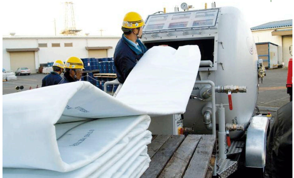
Above: Trelleborg epros drum, loading an inversion drum with a liner prior to installation
