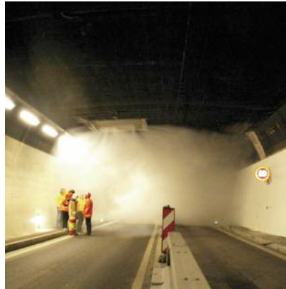
Above: Smoke extraction testing of the single-point smoke extractions system that replaced a distributed exhaust system in the single-tube Loppertunnel, Switzerland [Photo: HBI Haerter AG]
