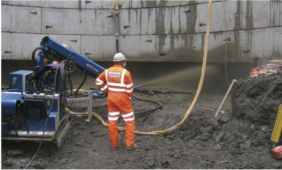
Above: SCL robot in operation during first SCL section of the HPOS
