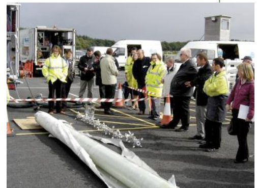
Above: Trelleborg epros drum, loading an inversion drum with a liner prior to installation
