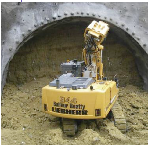
Above: Excavating underway under the canopy tubes
