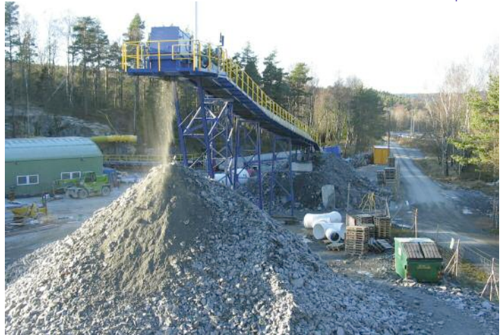
Right: The mucking belt delivers spoil
