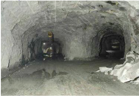
Above: The junction with the access tunnel
