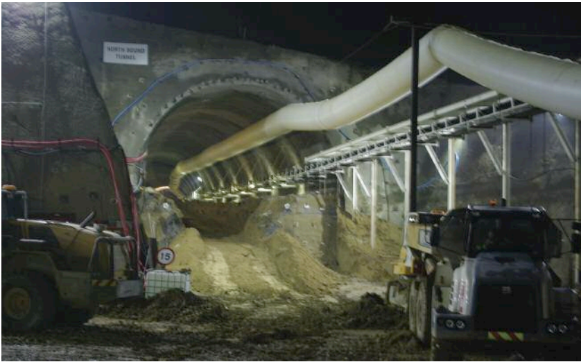
Above: Removal of muck via a belt conveyor
