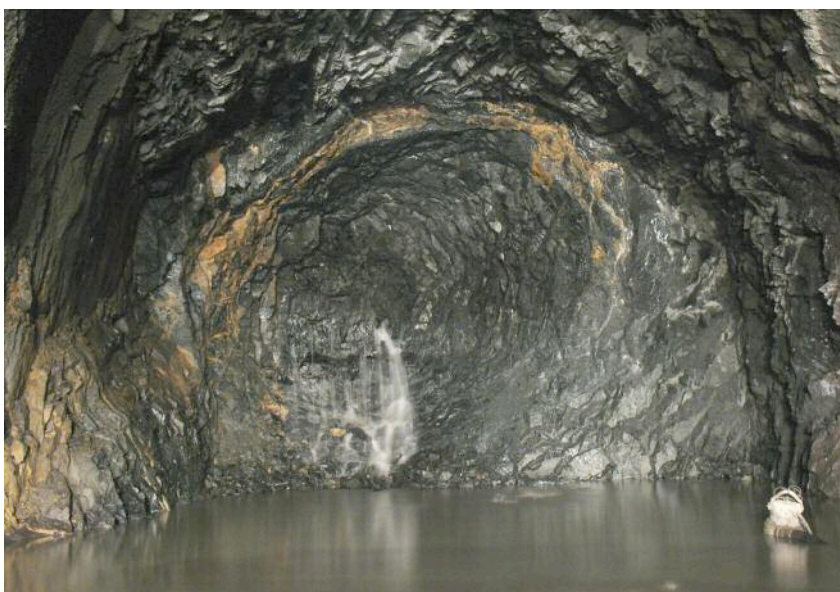
Left: Water at the face in the Siglufjörður tunnel
