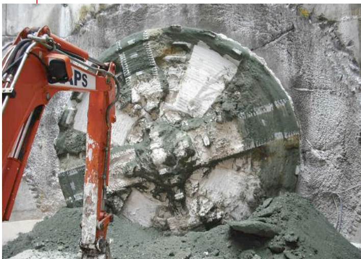
Above: Final breakthrough at Croydon Cable Tunnel, London
