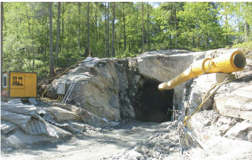
Above: The portal for the access tunnel
