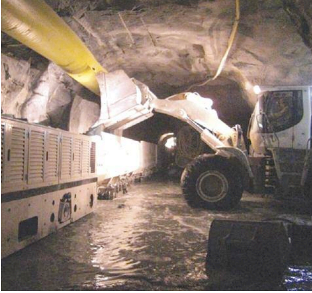
Above: Mucking onto the spoil train
