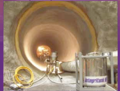
BORED TUNNELS SCL/NATM Construction
