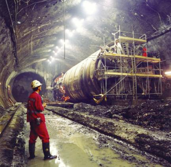
Above: The Channel Tunnel was a landmark project for Robbins
