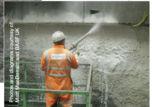
Above, left: Meyco Oruga in operation during the first SCL section of the shaft Above: Hand spraying the membrane
