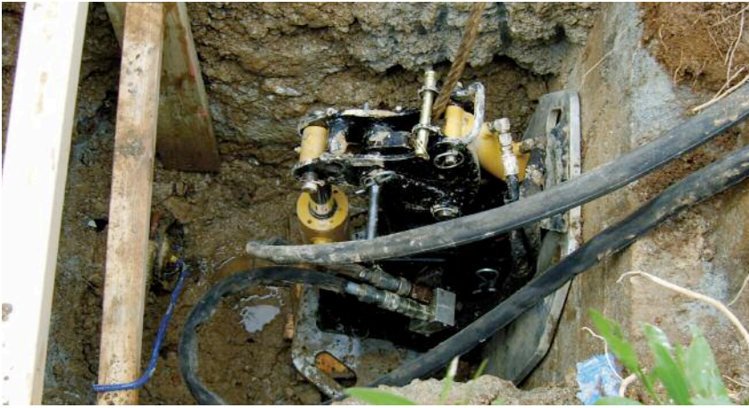
Above: A cable based, small footprint pipe burster set up for a bursting run in a small access pit (U Mole)
