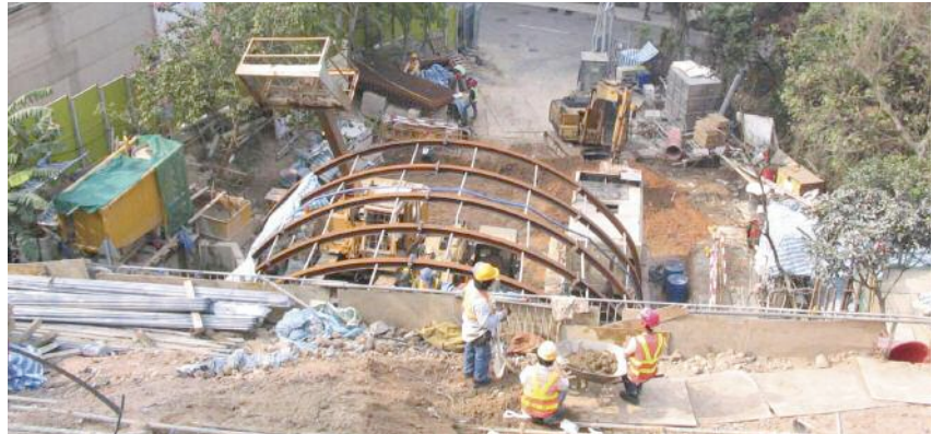
Above: The Po Shan Road Project utilised a Robbins 3.5m TBM launched from a confined 25m wide x 27m long jobsite
