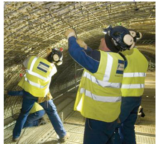
Top: Shotcreting; Bottom: Fixing and repairing the exposed lining rebar
