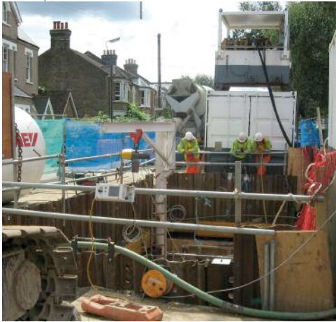
Above: The surface setup at the start shaft for the Sidcup drives Right: Holing on the first of the Sidcup drives
