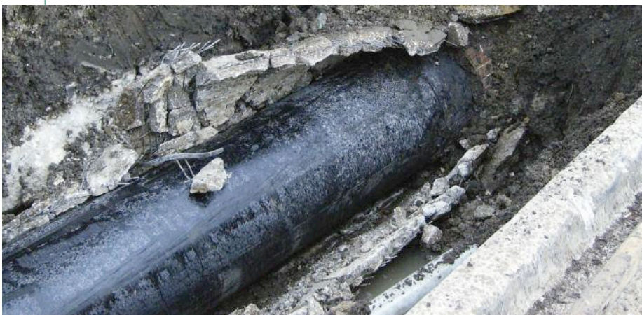
Below: A pneumatic pipe bursting unit bursting pipe (Hammerhead).
