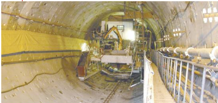
Left: Looking down the inclined bore at the Lovat TBM
