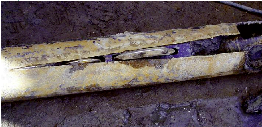
Below: A 'splitter' head cutting through the wall of a steel pipe (Hammerhead).
