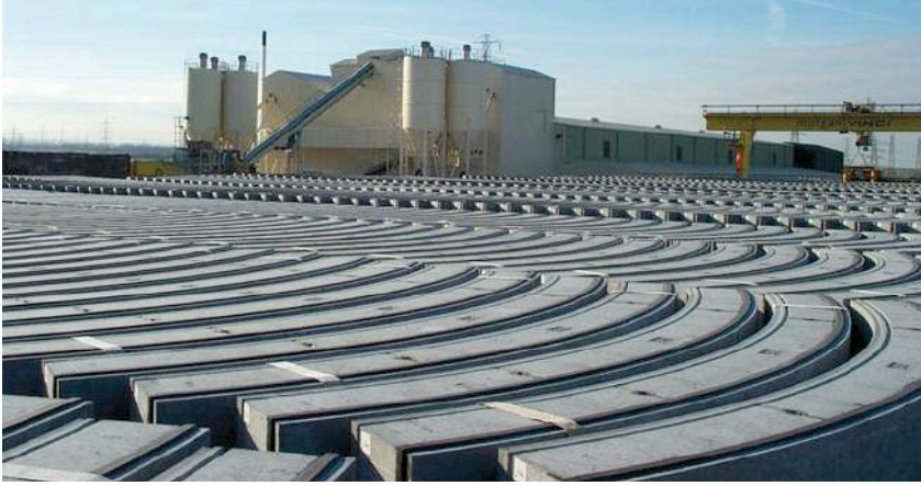
Above: A total of 44,500 precast segments have been required for the project
