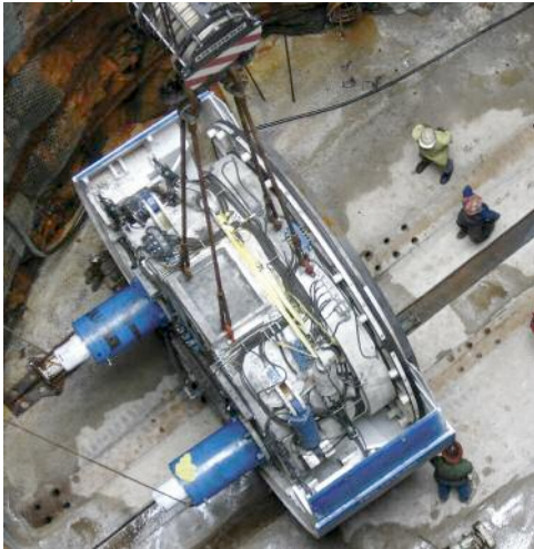
Above: The Robbins TBM at the Dobson's Run Project was launched from a shaft using umbilicals and 180-ton hydraulic jacks
