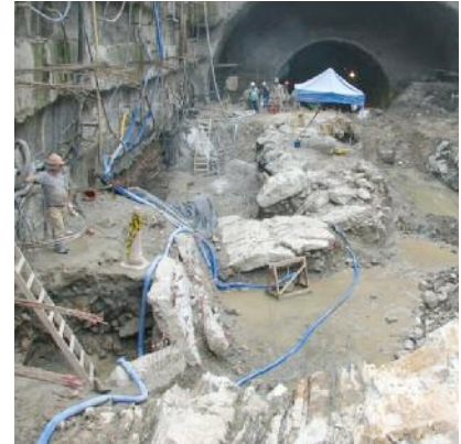
Left & below: Fig 7 - Sequence of the failure mechanism and construction debris during the archeological excavation
