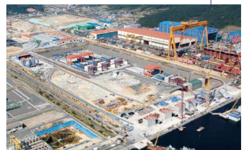
Below: Precast yard and model for fabrication of tunnel elements
