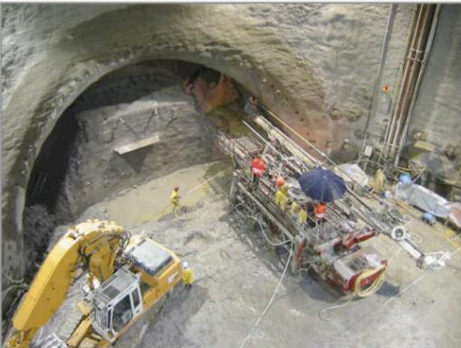
Olimpia Park North – Munich, Germany Underground railway, Lot 1 Forepoling
