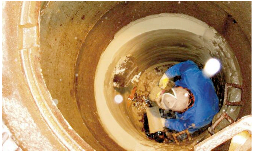
Above: Applying the ombran manhole rehabilitation system inside a manhole
