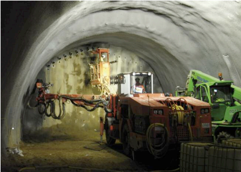
Above: Steel pipe canopy installation at weakest, south end of bores
