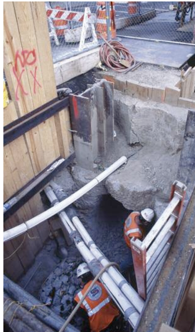
Above: Cramped working conditions above the alignment
