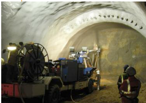
Above: Steel pipe canopy installation at weakest, south end of bores
