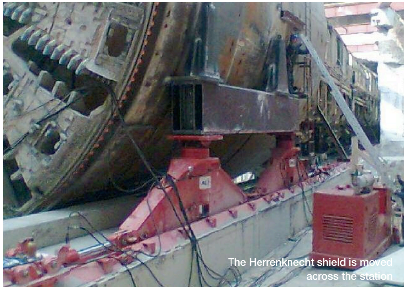
Fig 2: Sliding alignment for the TBM at Sagrera shaft
