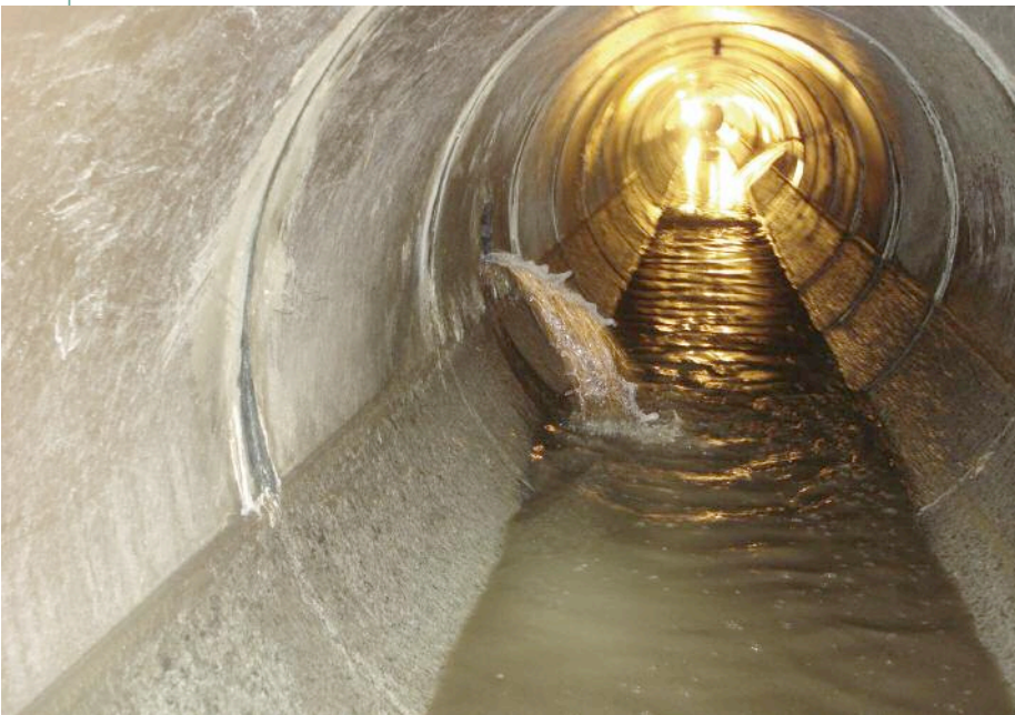
Below: The completed GRP liner with lateral connections reinstated
