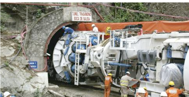
Above: The Robbins TBM being prepared for launch at Los Olmos
