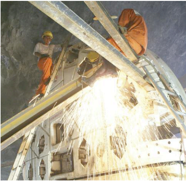
Above: The 5.3m diameter Robbins TBM assembly at Los Olmos, Peru; Right: The open shield was chosen due to high overburden
