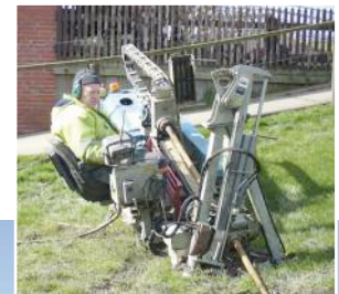
View of Oland and (inset) the Grundodrig 4X during a pilot bore
