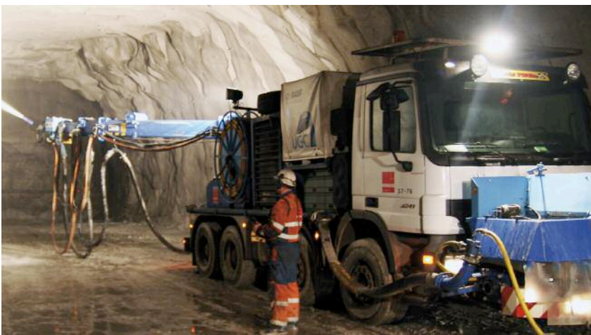
Above: BASF UGC's Roadrunner mechanised spraying equipment can be used for Masterseal waterproofing membrane application as well as shotcreting.
