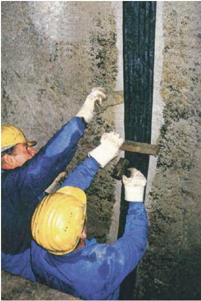
Above: Installing Phoenix drainage joint seals in the Dichtungen Tunnel
