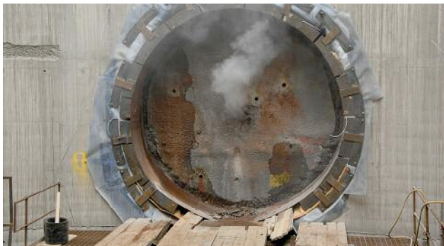
Morgan Est/Farrans JV holes through on Belfast Sewer
