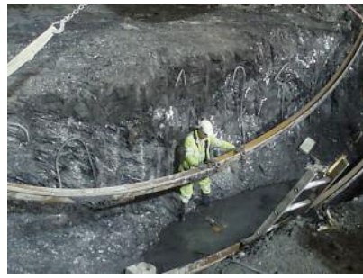
Above left: Installation of the highly deformable concrete elements in stage 2
