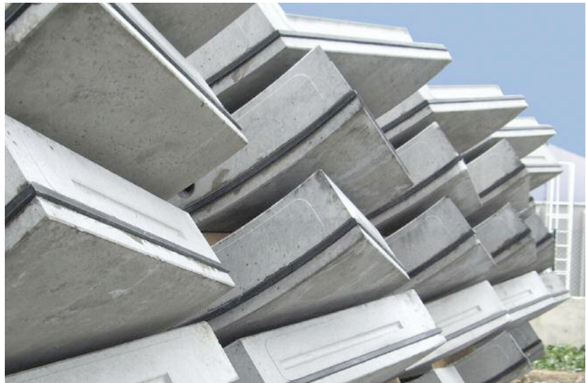
Above: Daetwyler Rubber CoexSwell segment gaskets with integral swelling compound used on pre-cast concrete waiting installation on the Marmaray Tunnel's bored section
