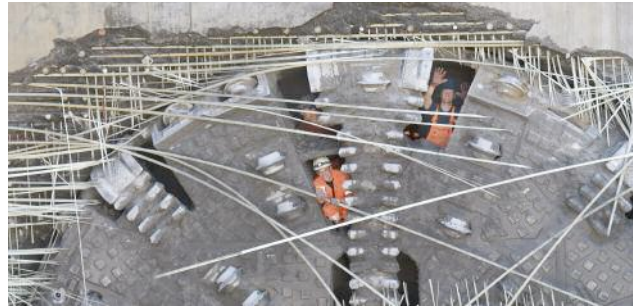
Left: Segments during construction of the Malmö Citytunnel Below: Final TBM breakthrough at Malmö C station
