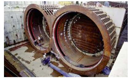
Above: TBM docking element on the immersed tube element
