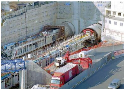
Above: The drive portal on the Asian side of the project
