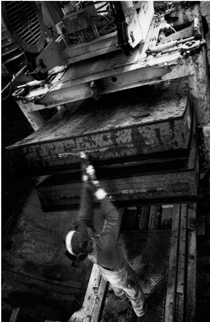
Left: Segments during construction of the Malmö Citytunnel Below: Final TBM breakthrough at Malmö C station
