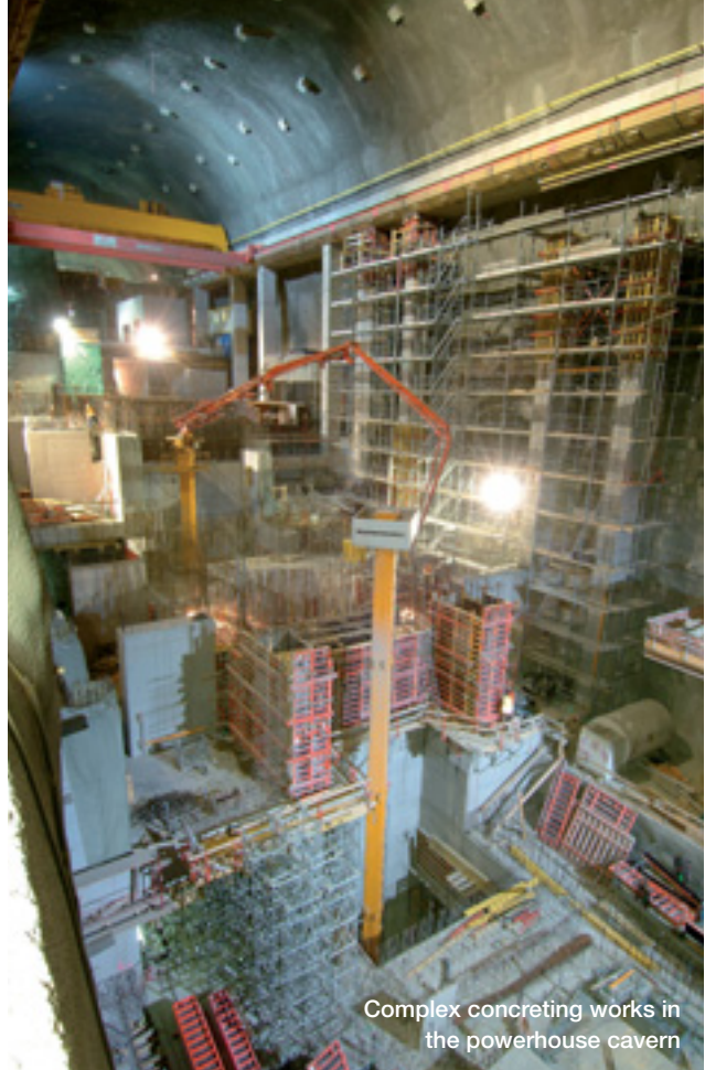
Pre-stressing of the strand anchors prior topheading pillar excavation
