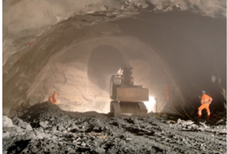
Above and left: Excavation of the powerhouse and transformer caverns proved particularly challenging
