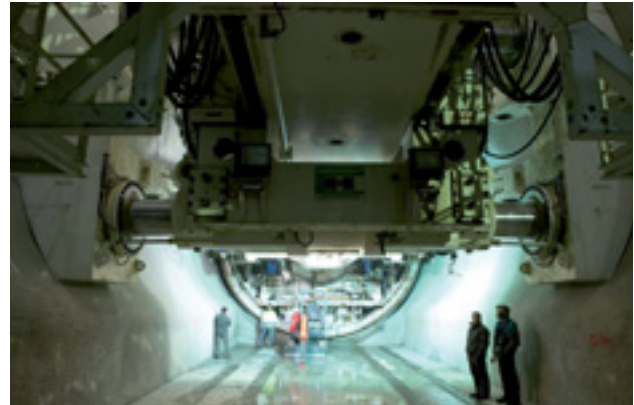
Grippers bracing walls at start of first Erstfeld drive at Gotthard
