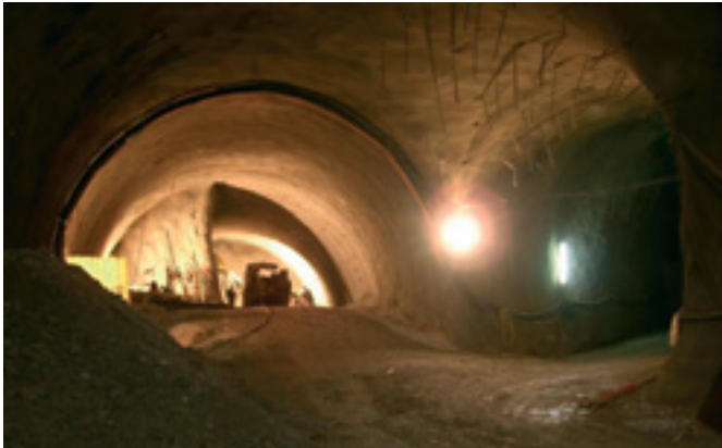
Above: Double-track top heading, bench and invert tunnelling
