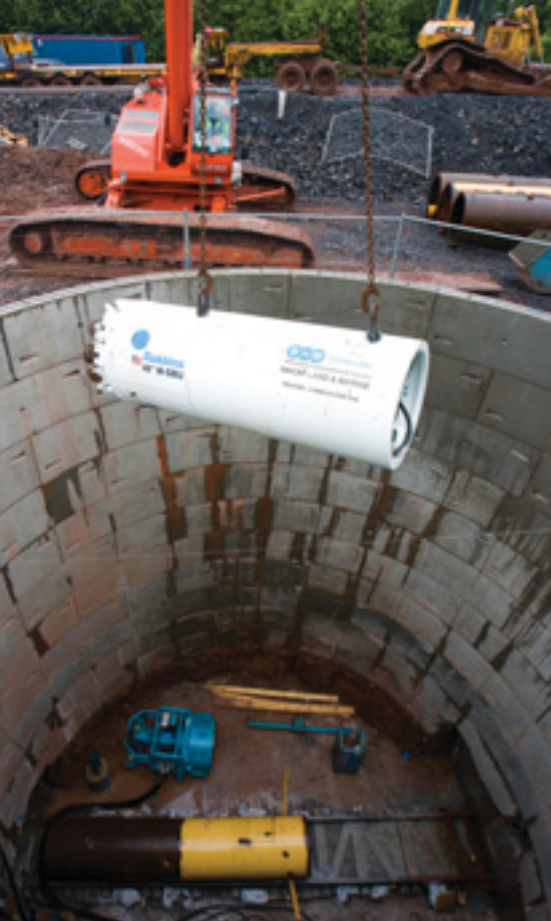
Above: A 1.2m Robbins SBU-M excavates a river crossing in siltstone between 70 and 200MPa
