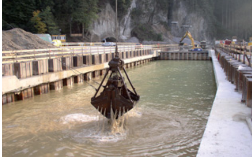
Above: Cells of sub-aqueous open cut construction below the high groundwater table on the H7 Fritzens-Baumkirchen
