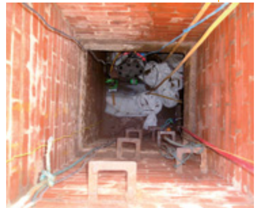
Above: Lining works underway
