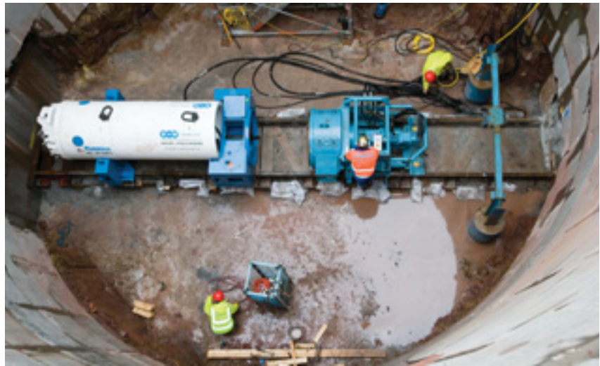
Above: A 1.2m Robbins SBU-M excavates a river crossing in siltstone between 70 and 200MPa
