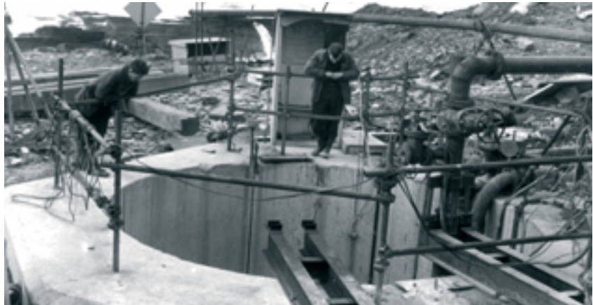
Above: Original shaft during construction
