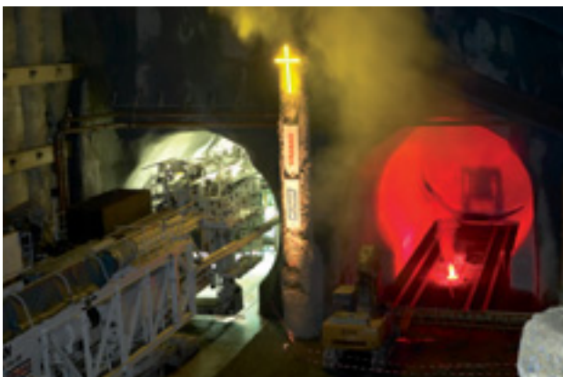
TBM launch on the Erstfeld section of the Gotthard Base Tunnel
