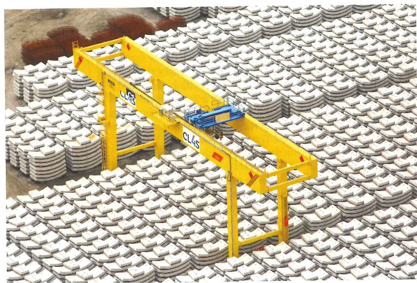
Above: Segment storage yard and gantry crane
