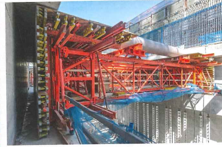
The VARIOKIT traveler system rolls from one section to the next on rails after each pour, without the formwork having to be broken down and reassembled.
