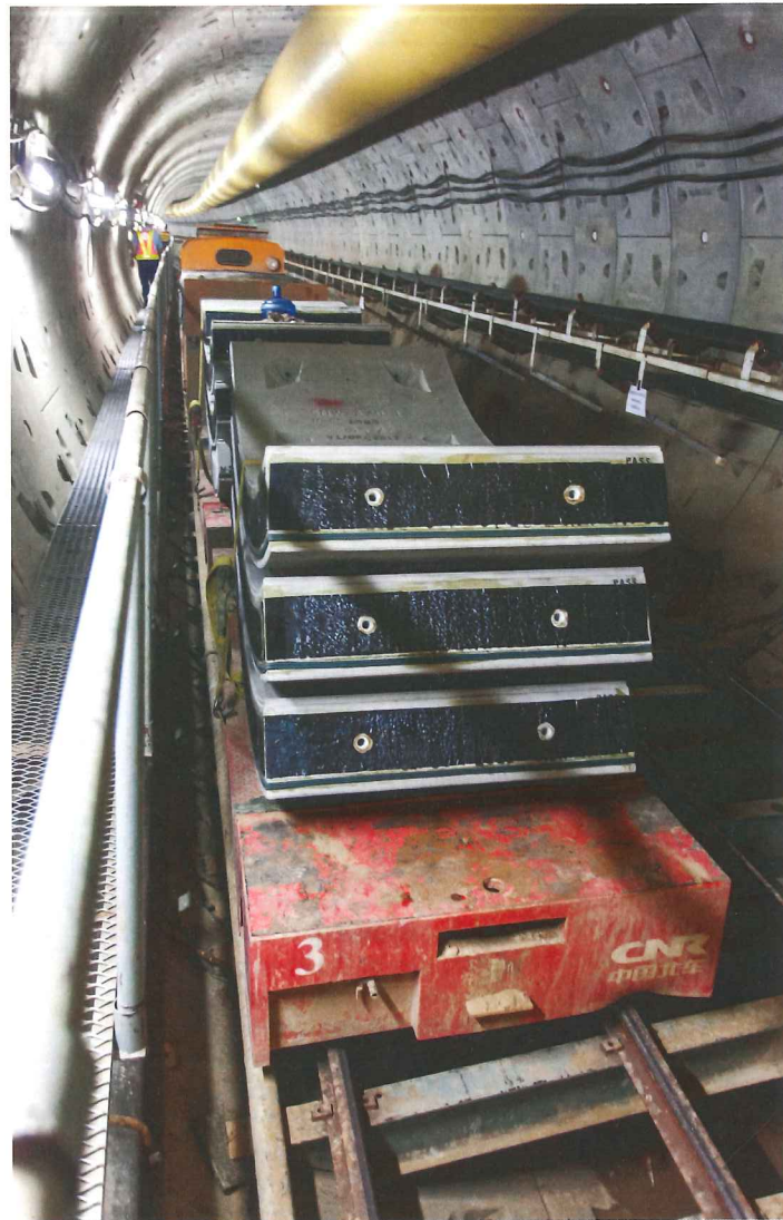
Above: Segments being transported to the TBM
