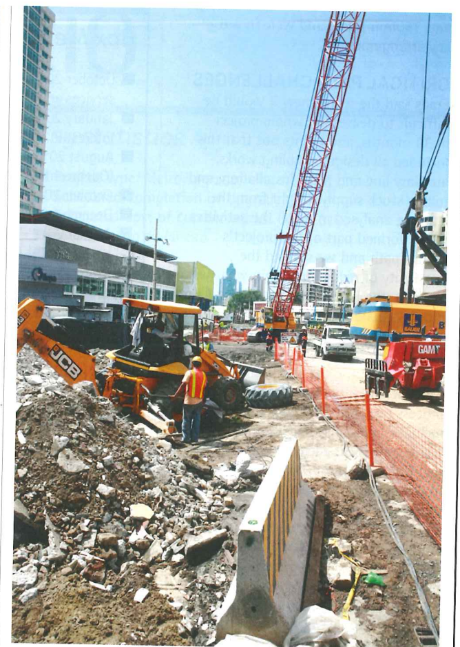
Above: Work ongoing in a congested site
