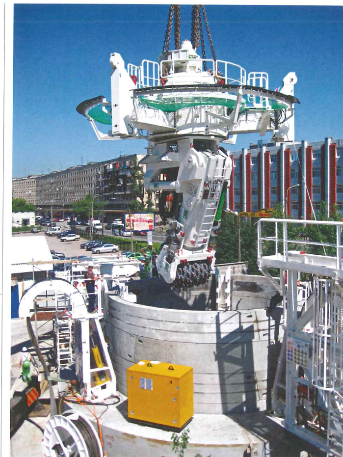
Above: Herrenknecht vertical borer on a metro ventilation shaft
