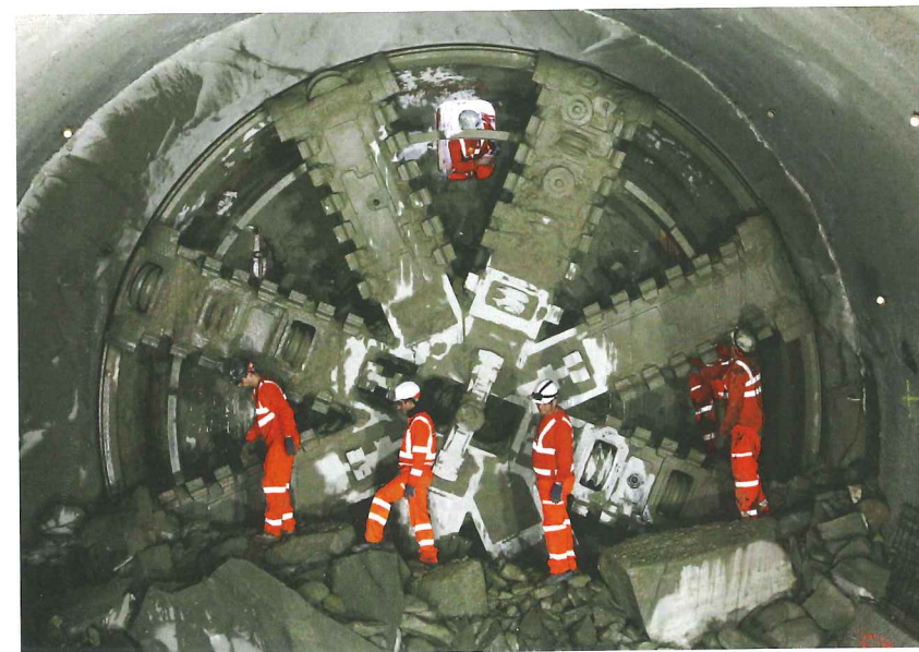
Below: TBM Elizabeth breaks through into Farringdon Station
