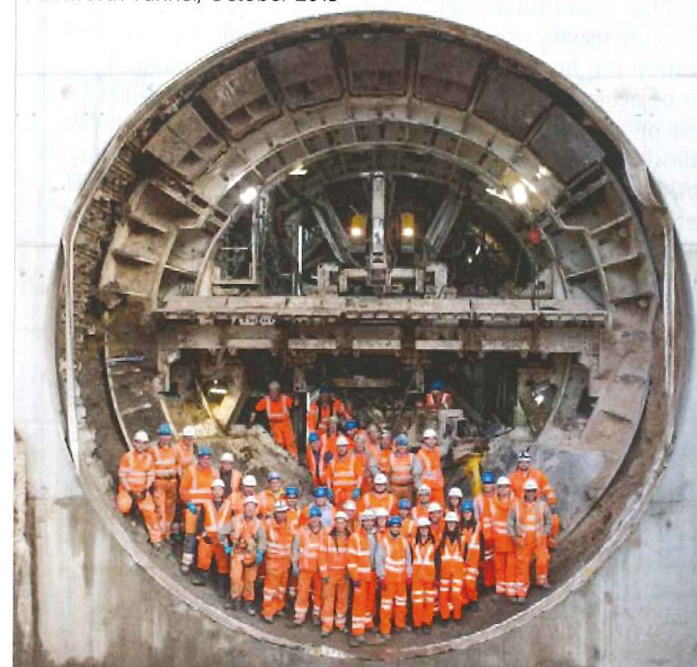
Specialists in underground design and supervision
