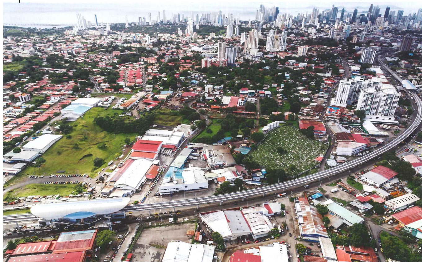
Below: An elevated section of the metro
