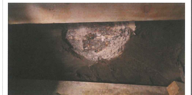
Above: Figure 16, A separation membrane was installed using a local breakout above the permanent works level. The work could be conducted under timber ensuring miners were not exposed to unsupported ground directly overhead
