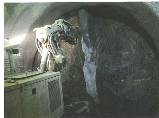
Right: Figure 13, Redundant pile encountered by Crossrail C300/C410 (BFK)
