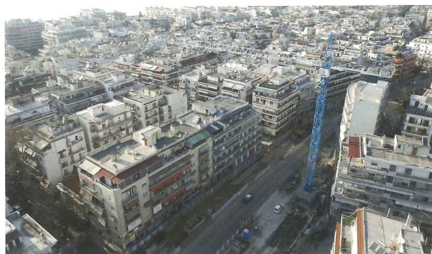
Both: Aerial view of lifting operations at two of the worksites
