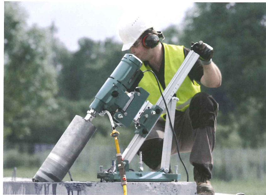
Above: Core-drilling operation ©VDMA
