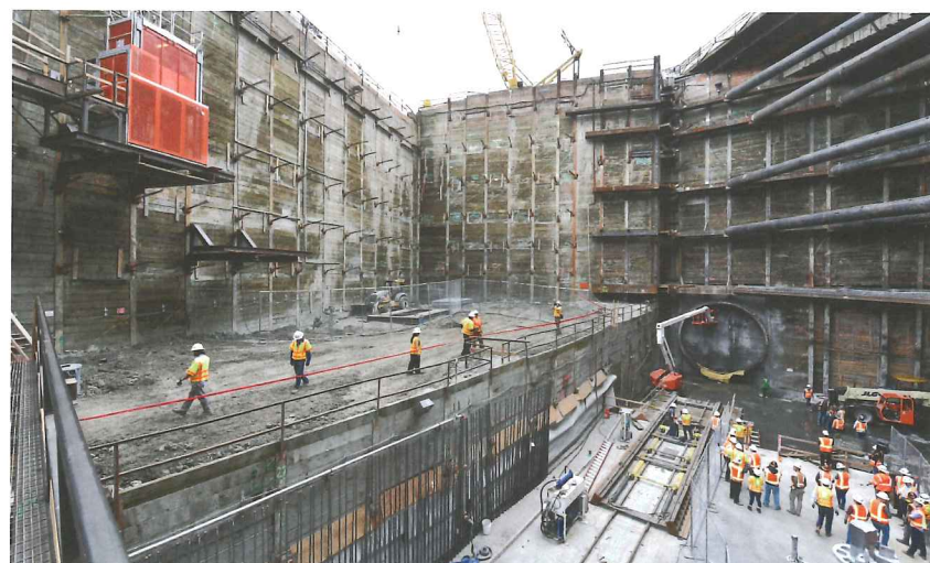
Above: Tunnel eye under construction on the Regional Connector project
