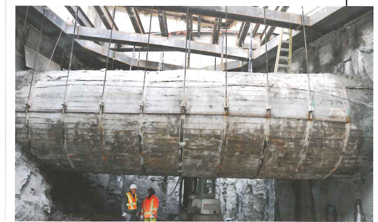
Below: The YDSS fully hanging across the connection chamber
