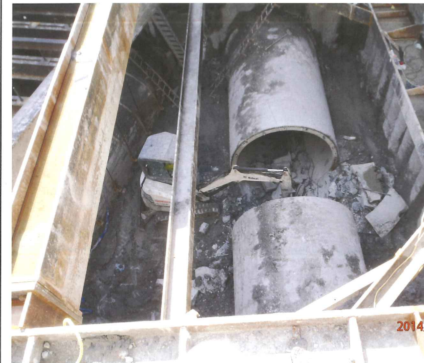
Above: Demolishing the SEC final lining
