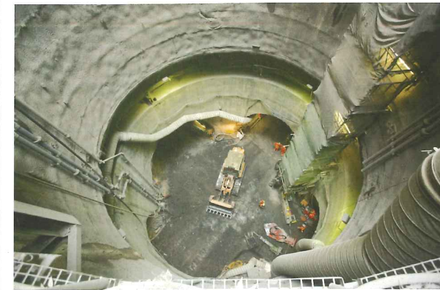
Left: Finsbury Circus shaft for Liverpool Street station and platform tunnels
