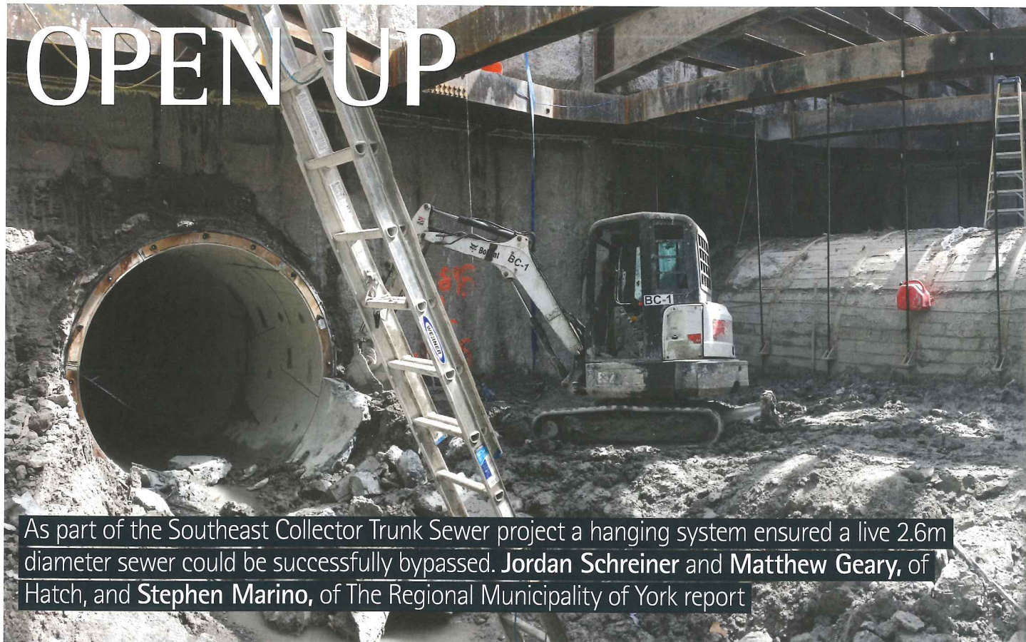
Above: The YDSS hanging system installed at springline and SEC PCTL demolished within the connection chamber
