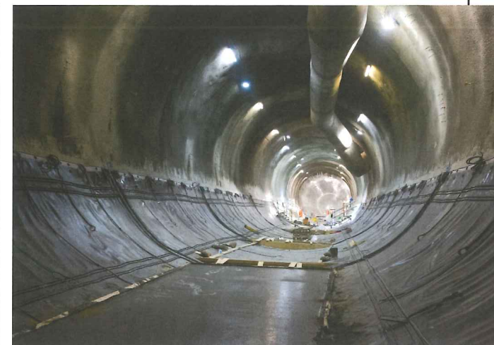
Above: Platform tunnel waterproofing lining works at Liverpool Street station
