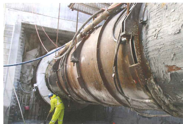
Right: Flume hanging system installed
