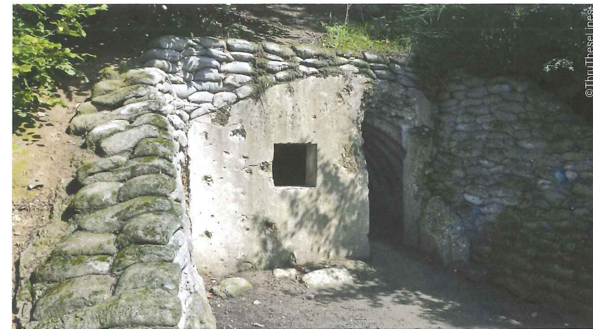
Above: The Lettenberg Bunkers on the Kemmelberg were built between April and May 1917 by the British Royal Engineers 175th Tunnelling Company. The five bunkers comprise a battalion headquarters, regimental aid post and troop accommodation beneath one of the most important observation view points from 1914, especially for the Messines Campaign of 1917. The bunkers are constructed of reinforced concrete poured in rough gravel on "elephant plates" - corrugated plates. Each bunker has an entrance and a window.
