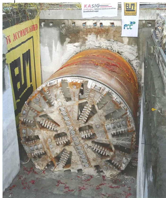
Above: The TBM breakthrough
