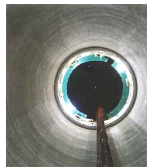
The Lee Tunnel shaft broke UK records for depth
