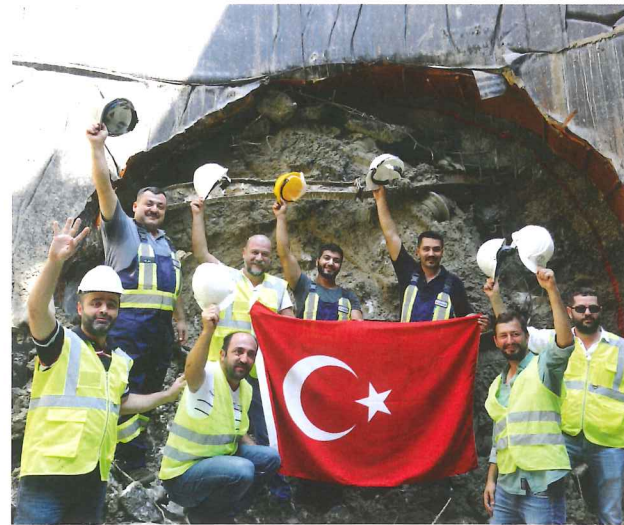
Breakthrough on the 3.91m-diameter sewer project
