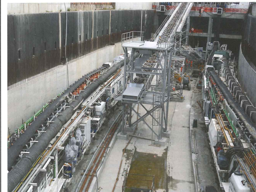
Above: The Sereni shaft is excavated in an open cut and it will be used as emergency exit and fire service access
