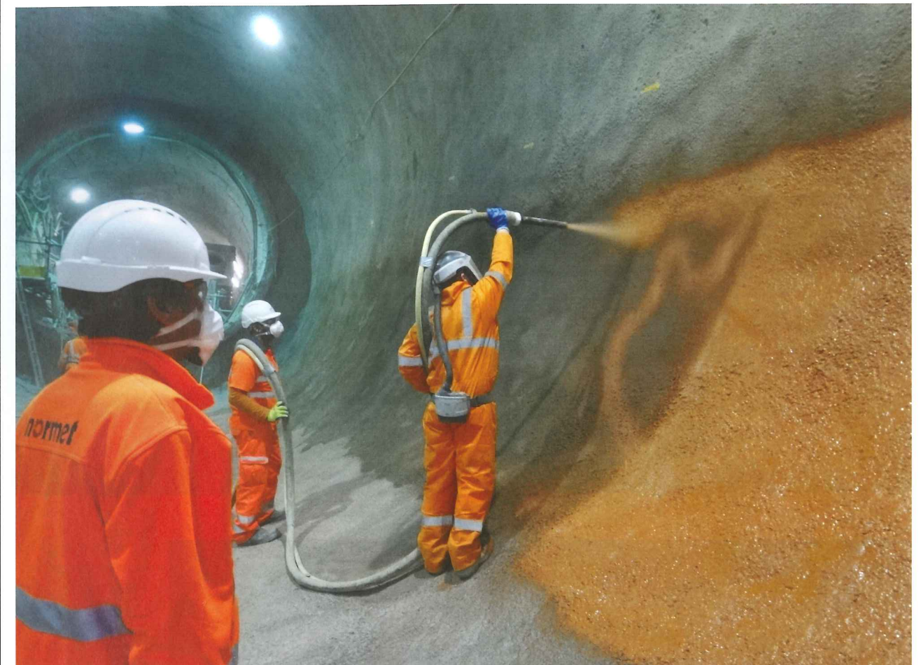
Above: Crossrail Fisher Street Cavern
