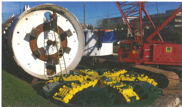
The TBM for the Northgate Link LRT project in Seattle
