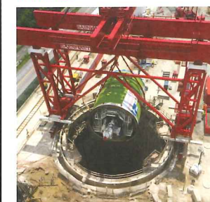
The TBM is lowered in D.C.
