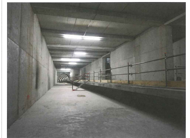
Below: The complete tunnel at the bottom of Forlanini FS railway
