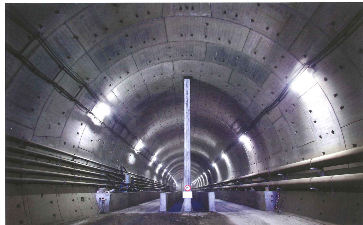
Below: The Green Heart Tunnel in the Netherlands, fully lined
