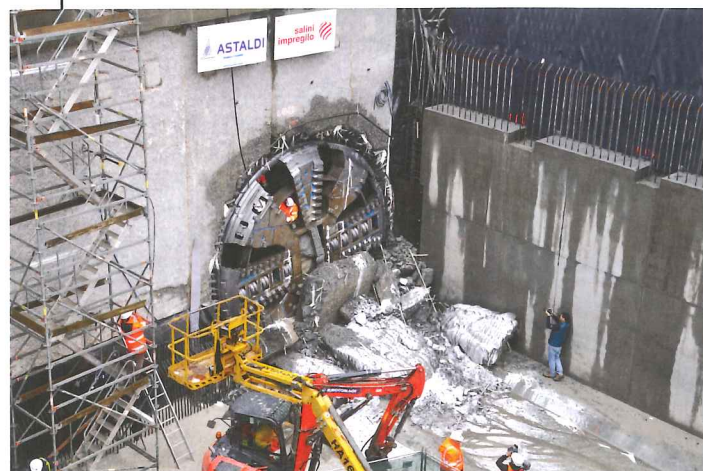
Above: TBM breakthrough
