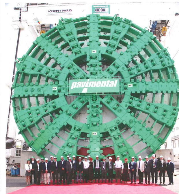
The Santa Lucia TBM in Schwanau, Germany
