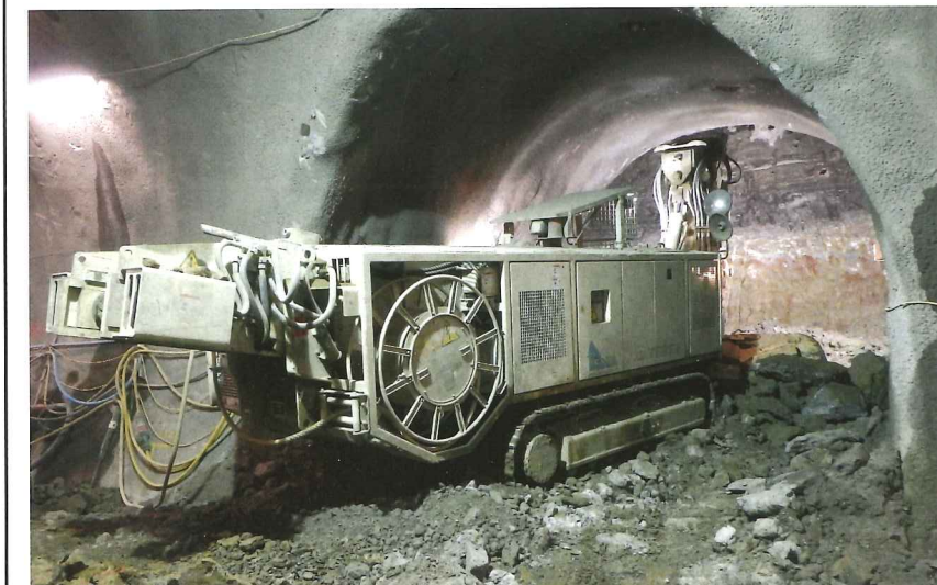
46 - Excavation at Farringdon Station, part of the Crossrail project
