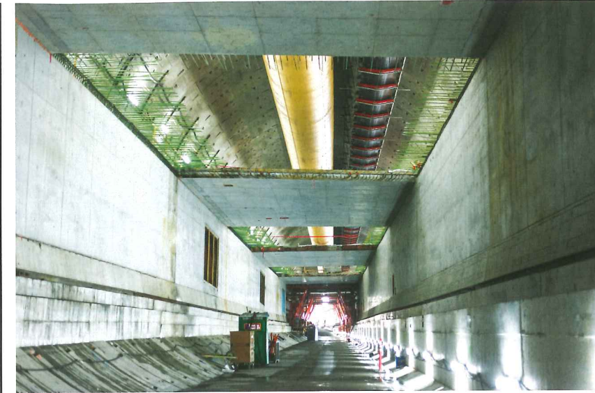
22 - The SR99 project in Seattle, Washington
